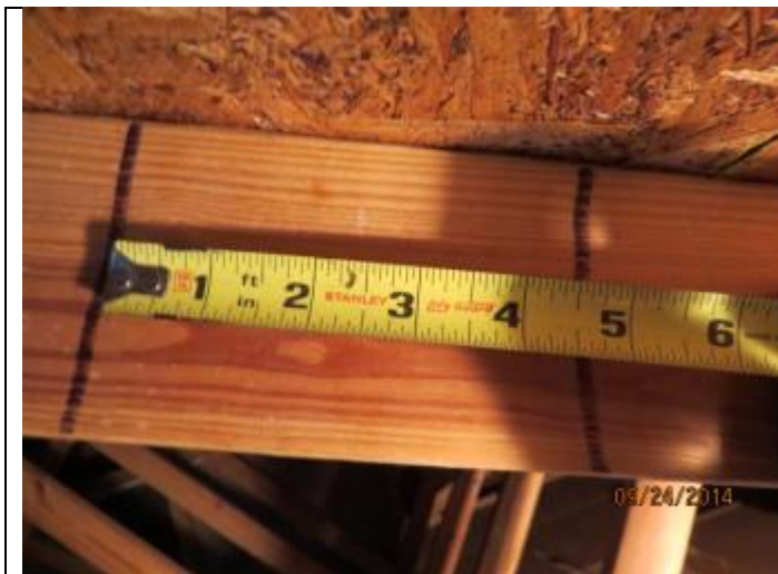
PHOTO 7 – Roof Deck Attachment Spacing
