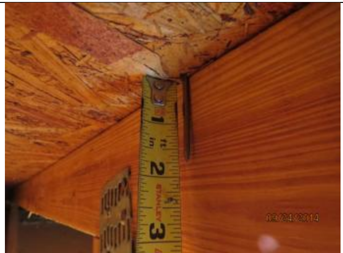
PHOTO 4 – Roof Deck Attachment = 8D Nails
