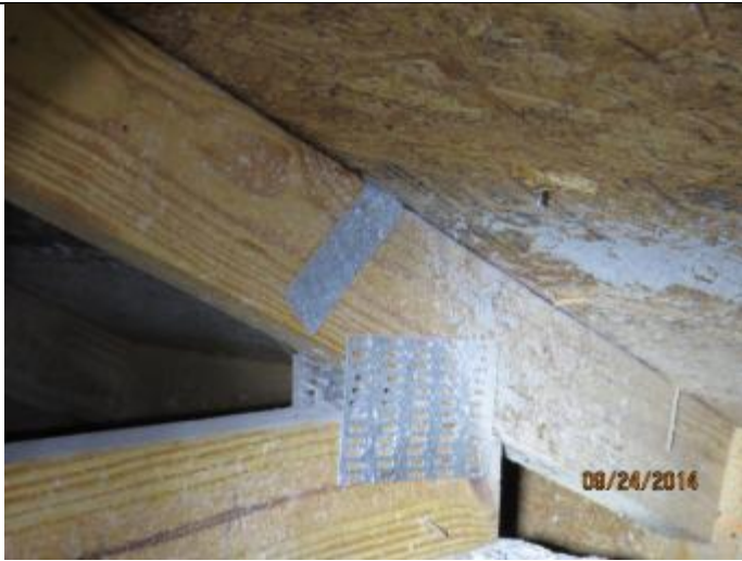
PHOTO 9 – Roof To Wall Attachment = Single Wrap Straps
