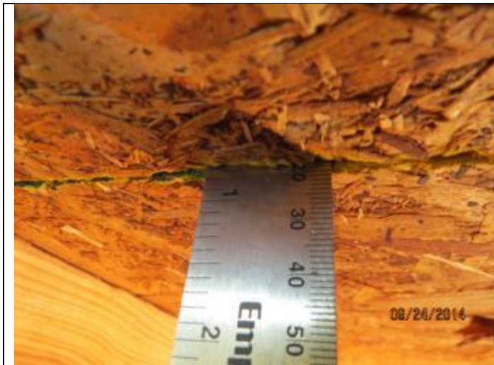
PHOTO 3 – Roof Deck = OSB
