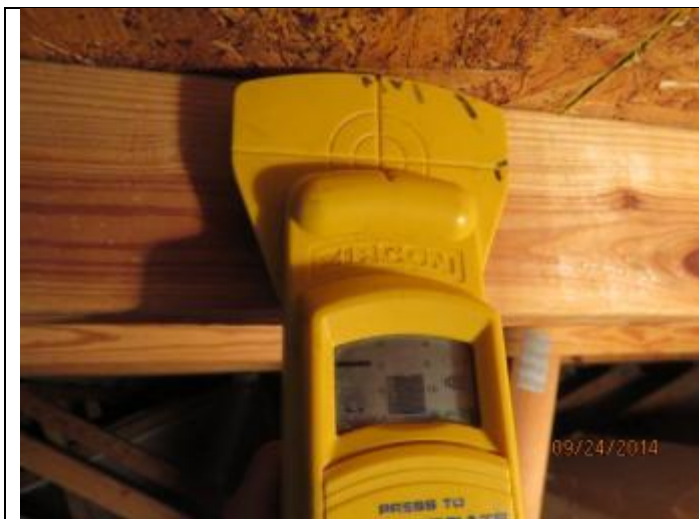
PHOTO 5 – Roof Deck Attachment Locations
