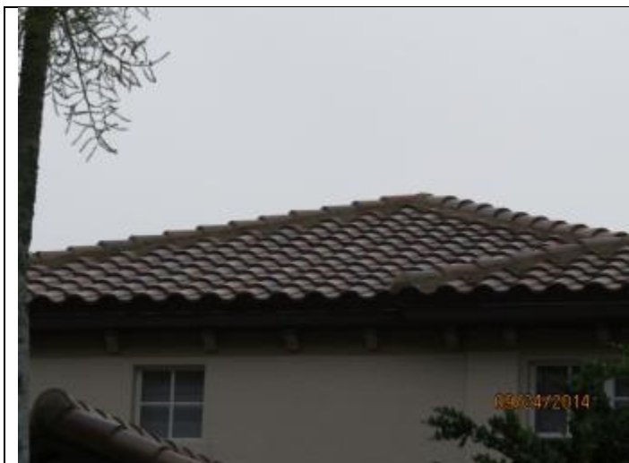
PHOTO 1 – Roof Overview, Covering = Tile
