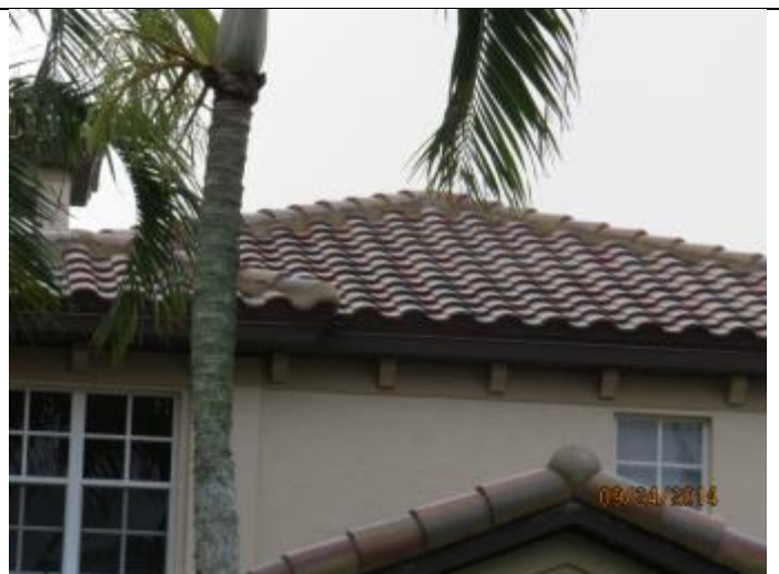
PHOTO 2 – Roof Overview, Covering = Tile
