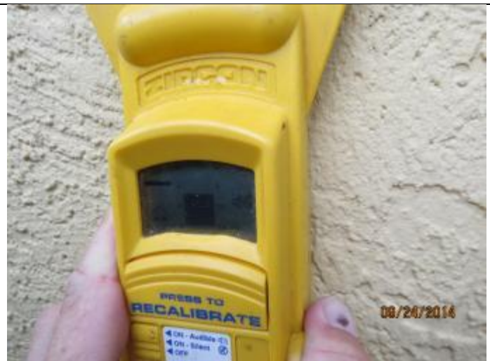
PHOTO 14 – Exterior Walls = Reinforced Masonry
