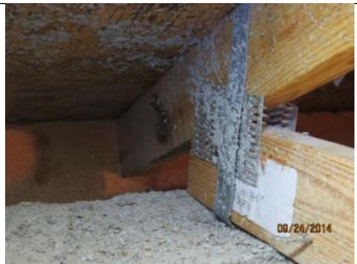
PHOTO 8 – Roof To Wall Attachment = Single Wrap Straps
