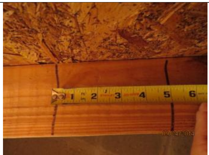
PHOTO 6 – Roof Deck Attachment Spacing
