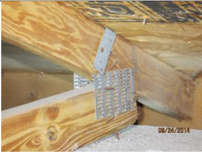
PHOTO 9 – Roof To Wall Attachment = Single Wrap Straps
