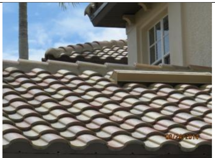
PHOTO 2 – Roof Overview, Covering = Tile
