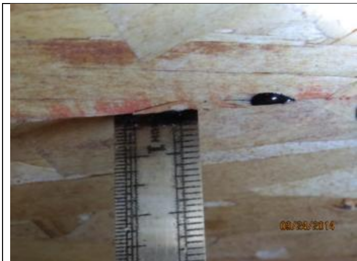
PHOTO 3 – Roof Deck = OSB
