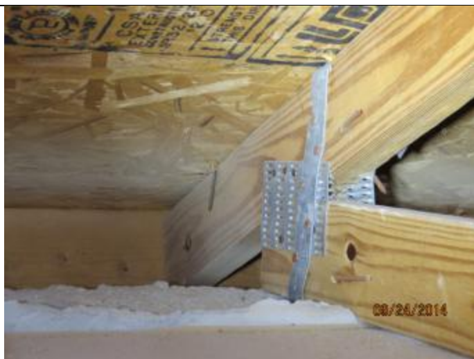
PHOTO 8 – Roof To Wall Attachment = Single Wrap Straps
