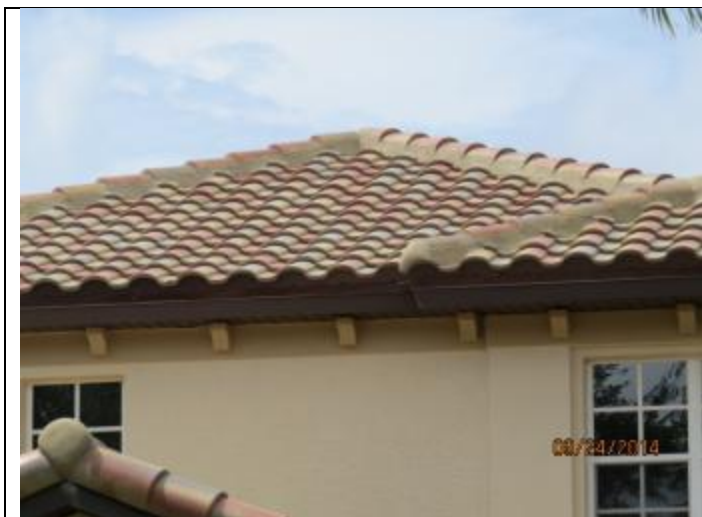
PHOTO 1 – Roof Overview, Covering = Tile
