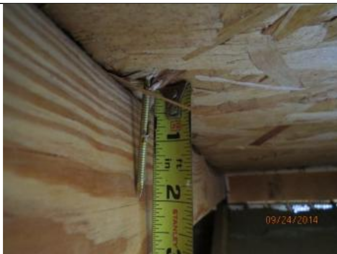
PHOTO 4 – Roof Deck Attachment = 8D Nails
