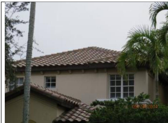
PHOTO 1 – Roof Overview, Covering = Tile
