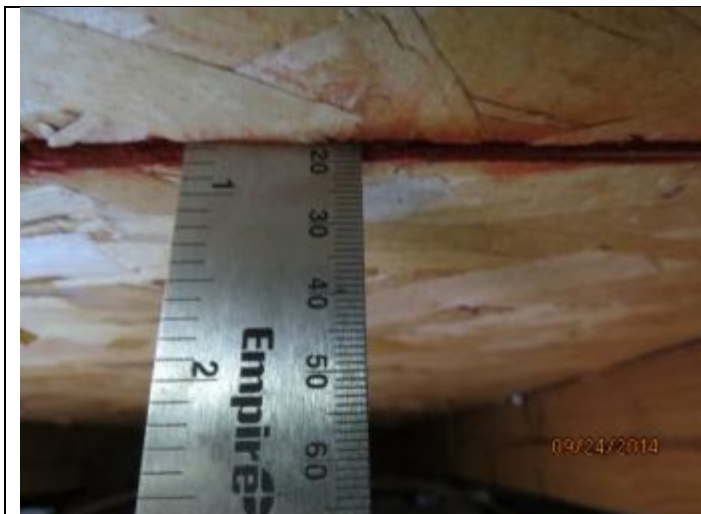
PHOTO 3 – Roof Deck = OSB
