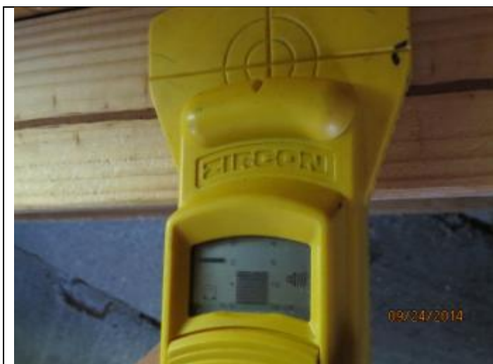
PHOTO 5 – Roof Deck Attachment Locations
