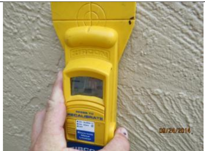
PHOTO 14 – Exterior Walls = Reinforced Masonry
