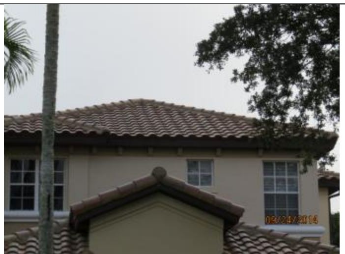
PHOTO 2 – Roof Overview, Covering = Tile
