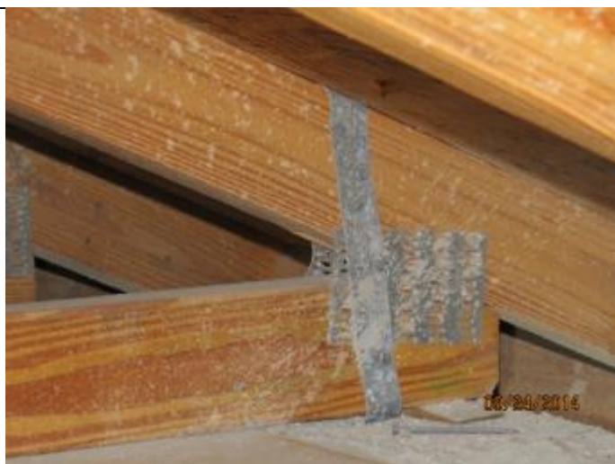
PHOTO 8 – Roof To Wall Attachment = Single Wrap Straps
