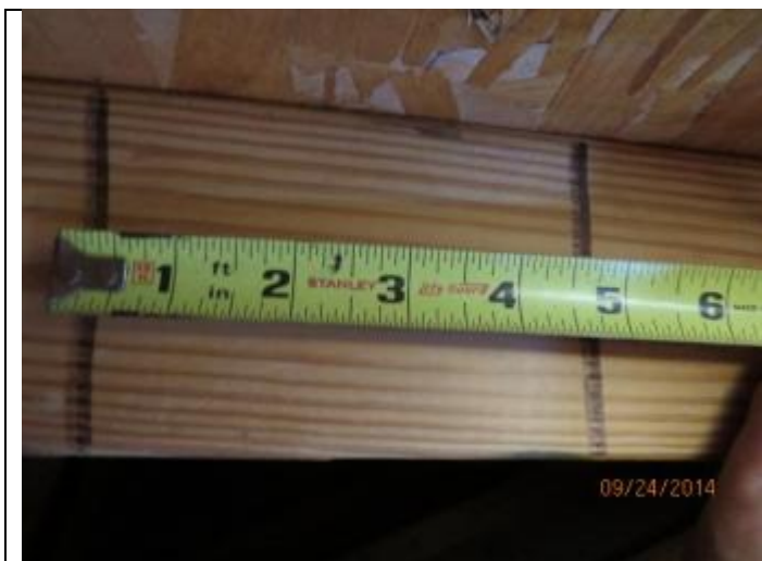
PHOTO 7 – Roof Deck Attachment Spacing
