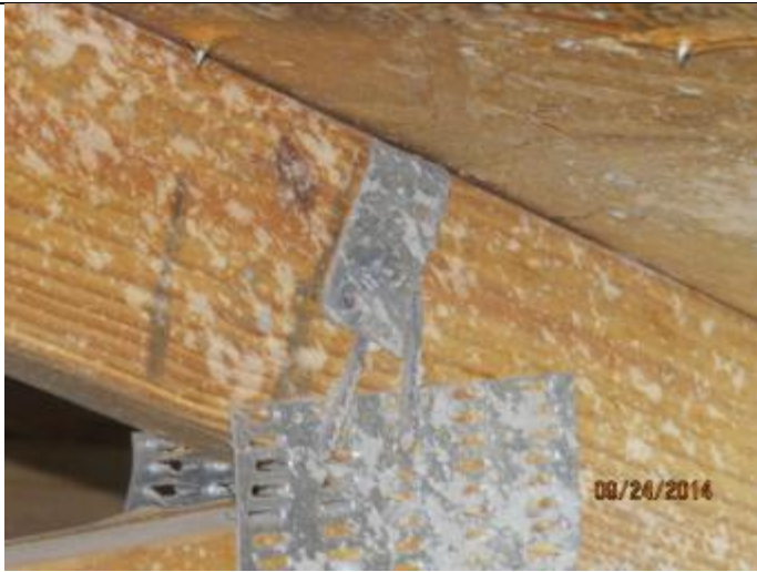
PHOTO 9 – Roof To Wall Attachment = Single Wrap Straps
