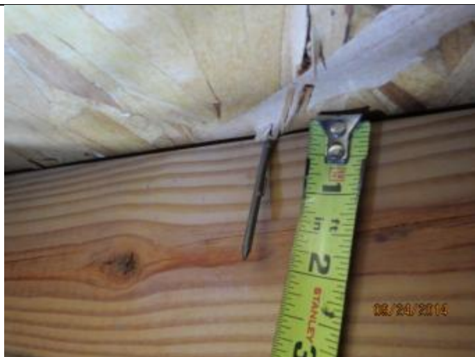
PHOTO 4 – Roof Deck Attachment = 8D Nails
