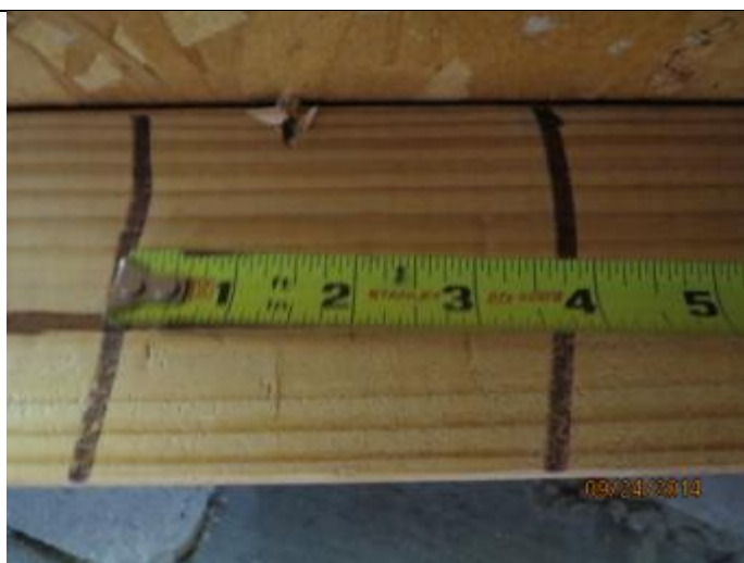
PHOTO 6 – Roof Deck Attachment Spacing
