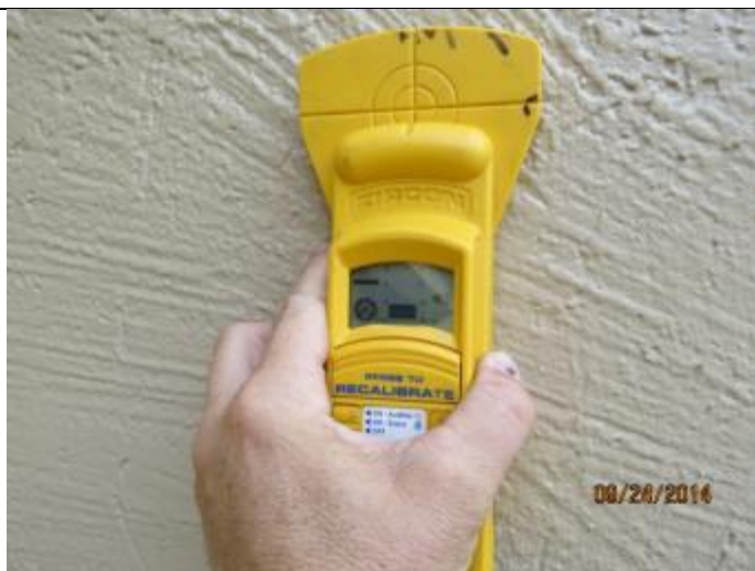
PHOTO 14 – Exterior Walls = Reinforced Masonry
