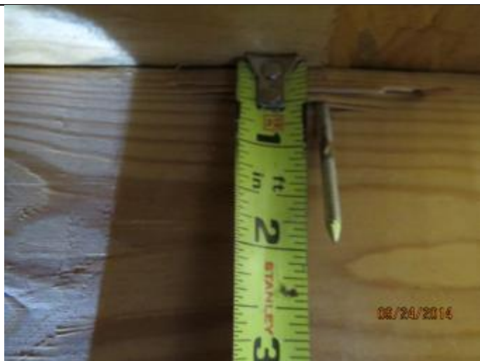
PHOTO 4 – Roof Deck Attachment = 8D Nails
