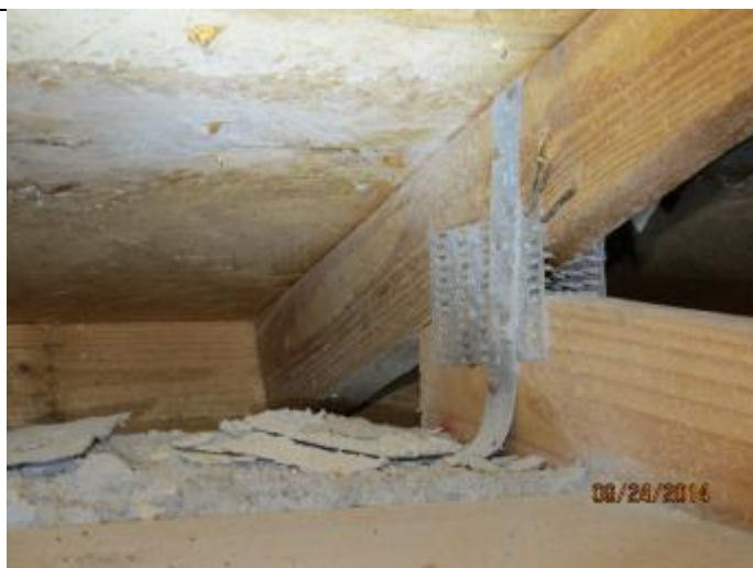
PHOTO 8 – Roof To Wall Attachment = Single Wrap Straps
