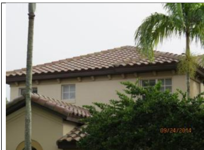
PHOTO 1 – Roof Overview, Covering = Tile
