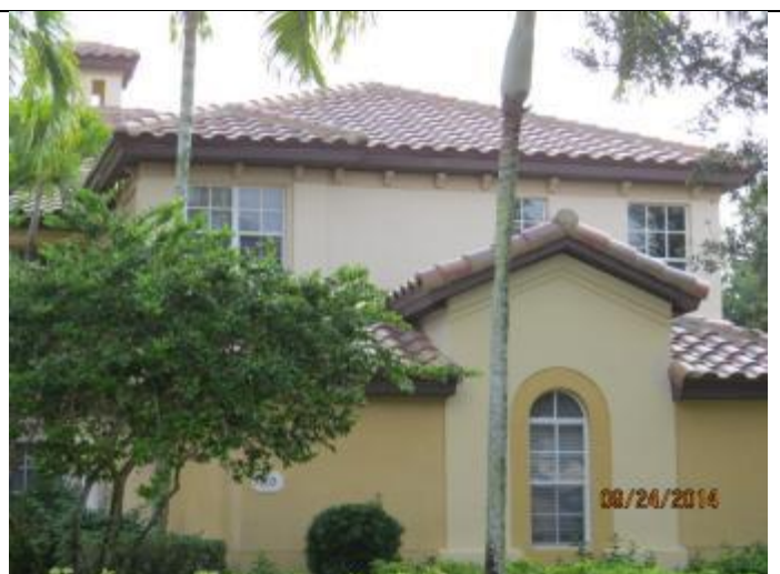
PHOTO 2 – Roof Overview, Covering = Tile
