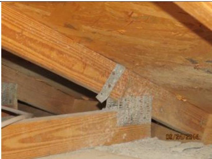
PHOTO 9 – Roof To Wall Attachment = Single Wrap Straps
