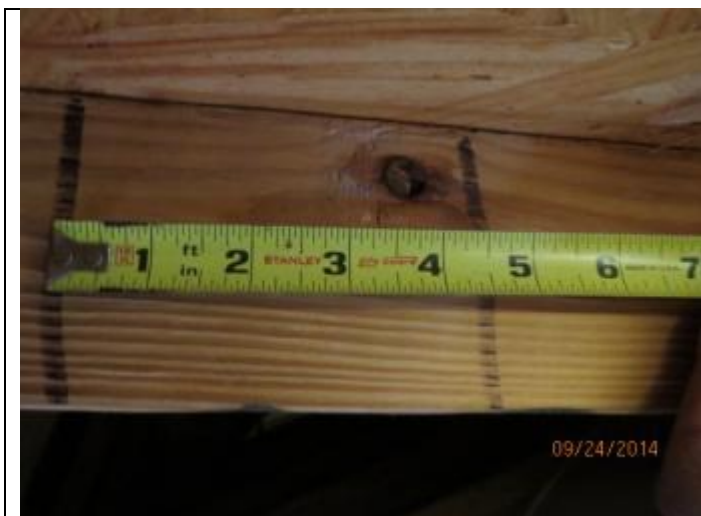
PHOTO 7 – Roof Deck Attachment Spacing
