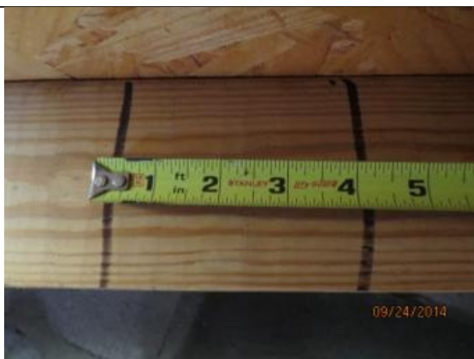
PHOTO 6 – Roof Deck Attachment Spacing
