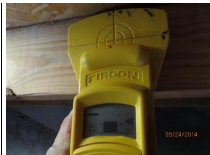
PHOTO 5 – Roof Deck Attachment Locations
