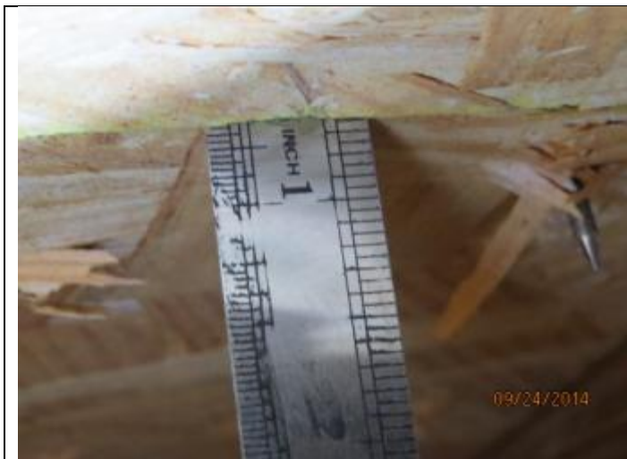
PHOTO 3 – Roof Deck = OSB
