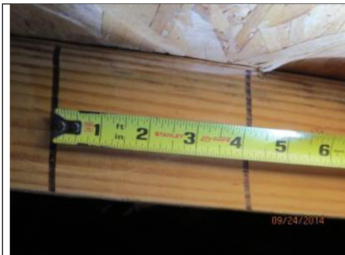
PHOTO 7 – Roof Deck Attachment Spacing
