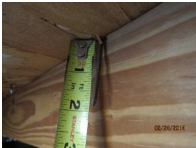
PHOTO 4 – Roof Deck Attachment = 8D Nails
