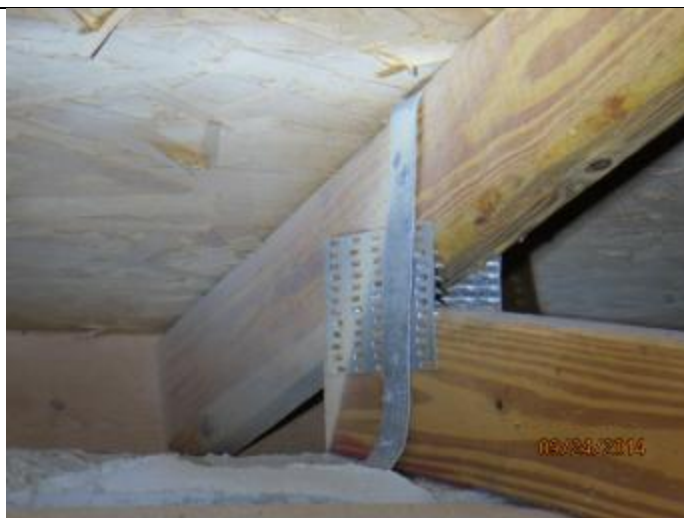
PHOTO 8 – Roof To Wall Attachment = Single Wrap Straps
