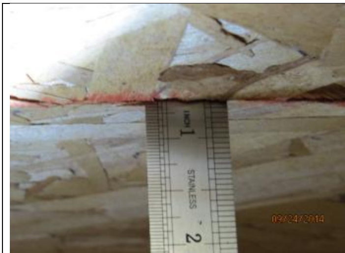
PHOTO 3 – Roof Deck = OSB
