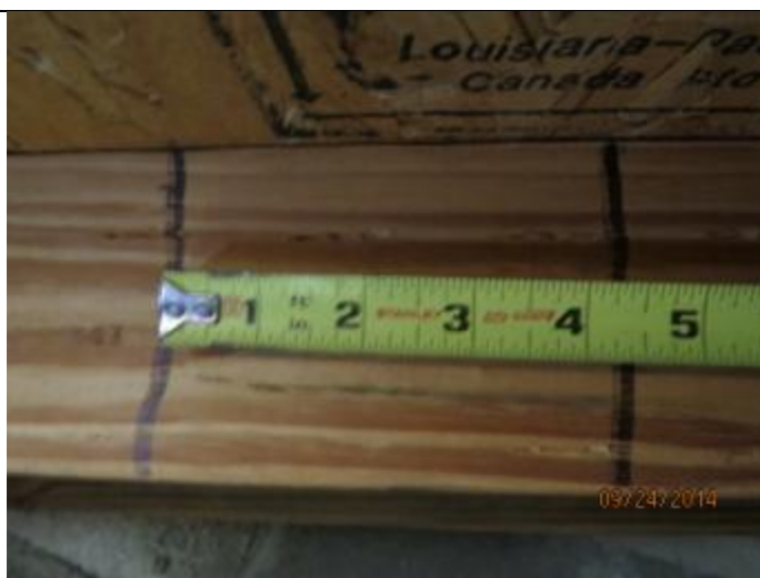
PHOTO 6 – Roof Deck Attachment Spacing
