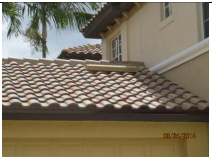
PHOTO 2 – Roof Overview, Covering = Tile
