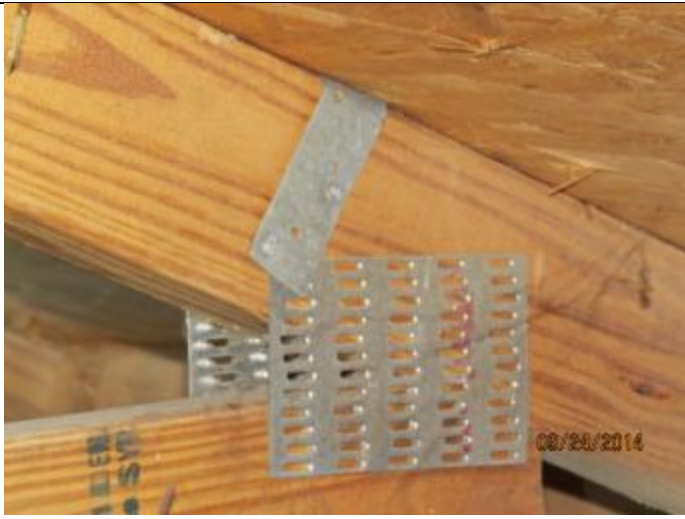
PHOTO 9 – Roof To Wall Attachment = Single Wrap Straps
