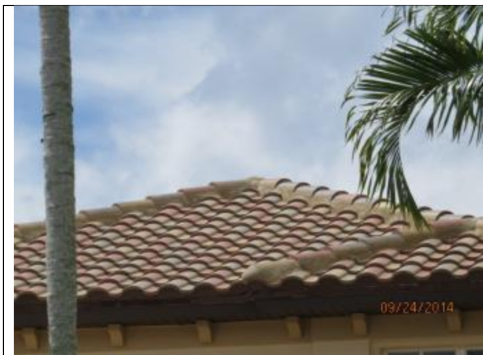
PHOTO 1 – Roof Overview, Covering = Tile
