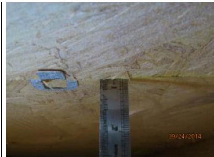
PHOTO 3 – Roof Deck = OSB
