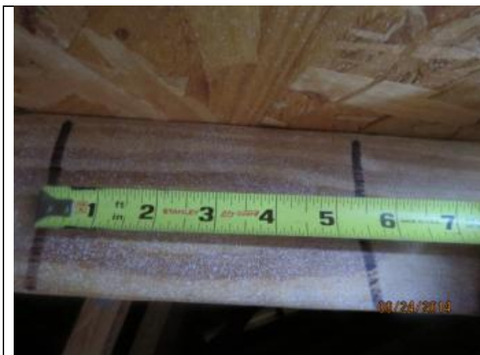
PHOTO 7 – Roof Deck Attachment Spacing
