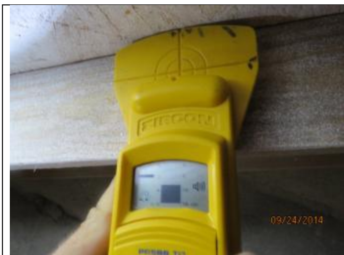
PHOTO 5 – Roof Deck Attachment Locations
