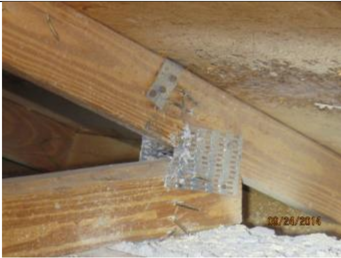
PHOTO 9 – Roof To Wall Attachment = Single Wrap Straps
