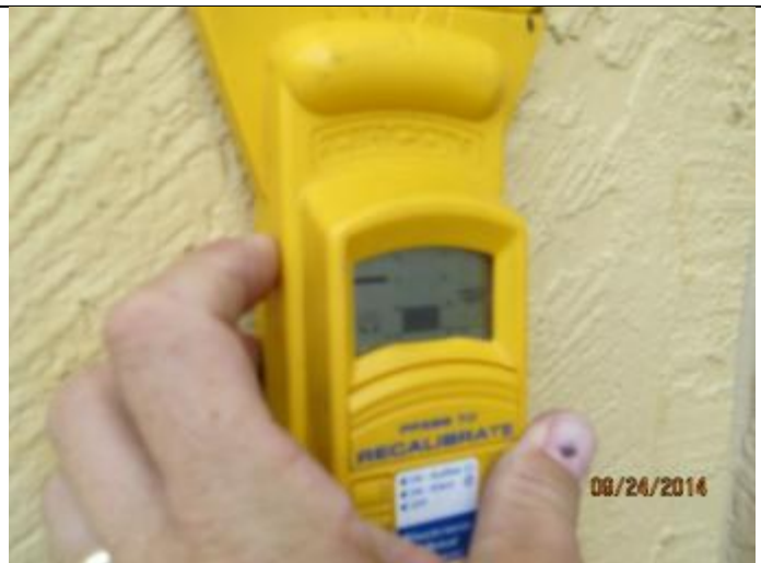
PHOTO 14 – Exterior Walls = Reinforced Masonry
