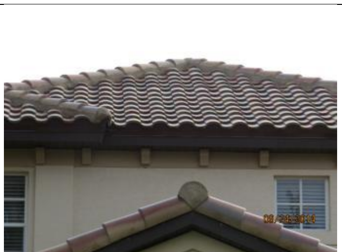
PHOTO 2 – Roof Overview, Covering = Tile
