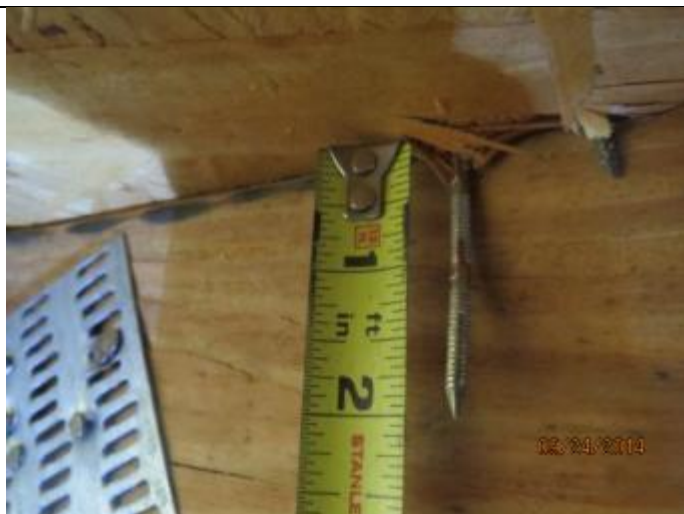
PHOTO 4 – Roof Deck Attachment = 8D Nails
