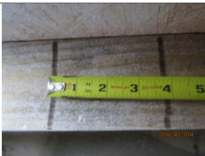
PHOTO 6 – Roof Deck Attachment Spacing
