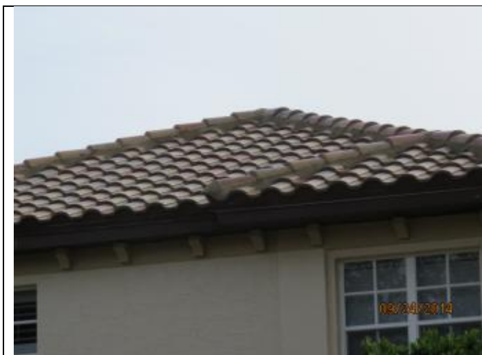
PHOTO 1 – Roof Overview, Covering = Tile
