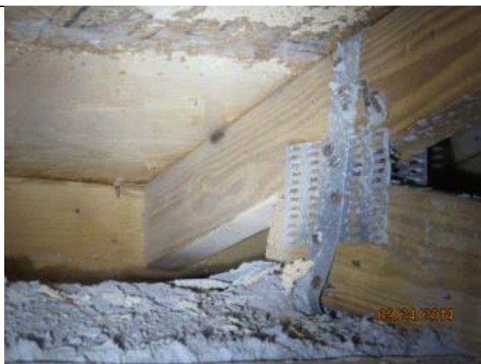
PHOTO 8 – Roof To Wall Attachment = Single Wrap Straps
