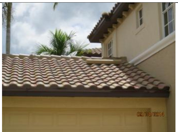
PHOTO 2 – Roof Overview, Covering = Tile
