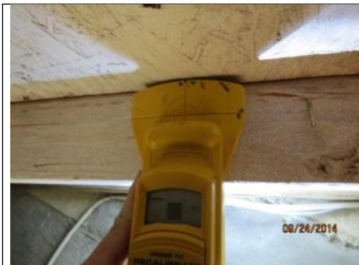
PHOTO 5 – Roof Deck Attachment Locations
