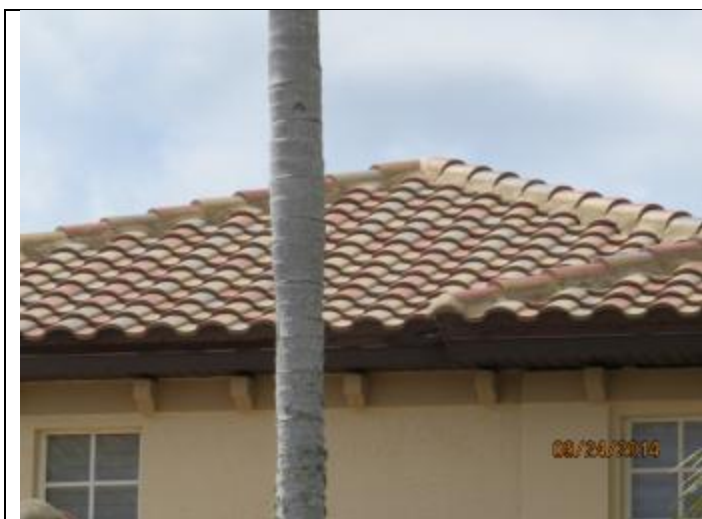
PHOTO 1 – Roof Overview, Covering = Tile
