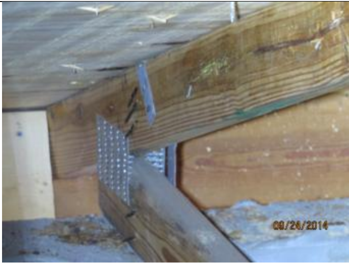
PHOTO 9 – Roof To Wall Attachment = Single Wrap Straps
