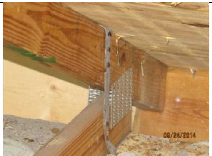
PHOTO 8 – Roof To Wall Attachment = Single Wrap Straps
