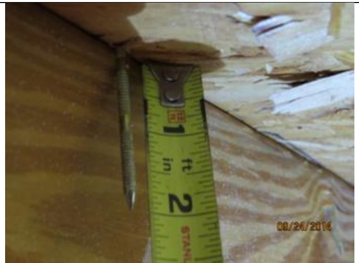
PHOTO 4 – Roof Deck Attachment = 8D Nails
