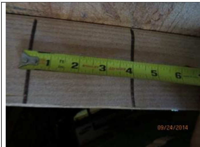
PHOTO 7 – Roof Deck Attachment Spacing
