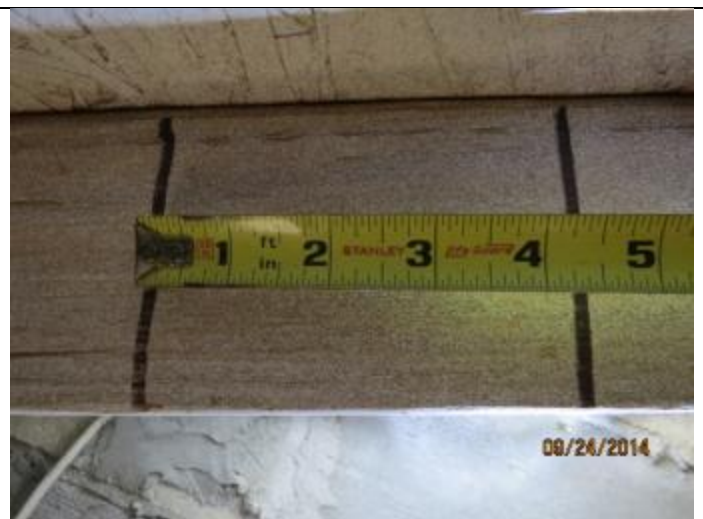
PHOTO 6 – Roof Deck Attachment Spacing
