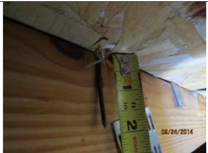
PHOTO 4 – Roof Deck Attachment = 8D Nails
