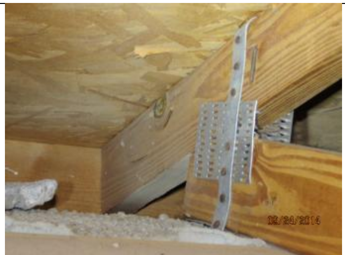
PHOTO 8 – Roof To Wall Attachment = Single Wrap Straps
