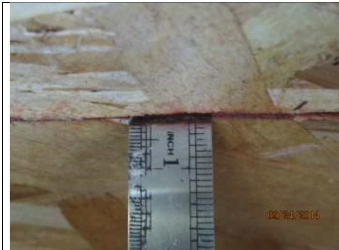
PHOTO 3 – Roof Deck = OSB
