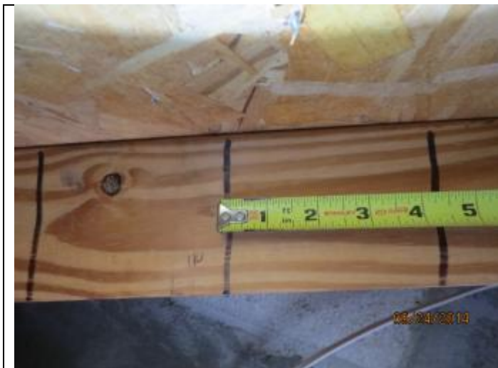
PHOTO 7 – Roof Deck Attachment Spacing
