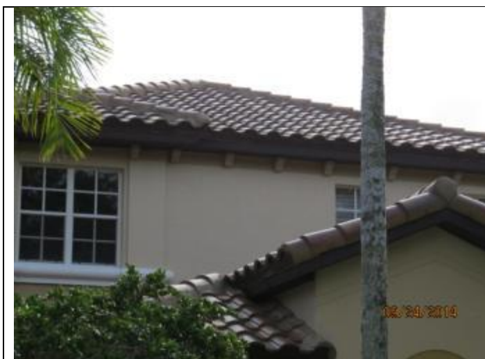
PHOTO 1 – Roof Overview, Covering = Tile
