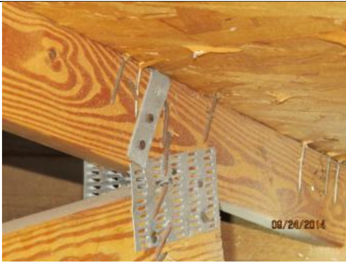
PHOTO 9 – Roof To Wall Attachment = Single Wrap Straps
