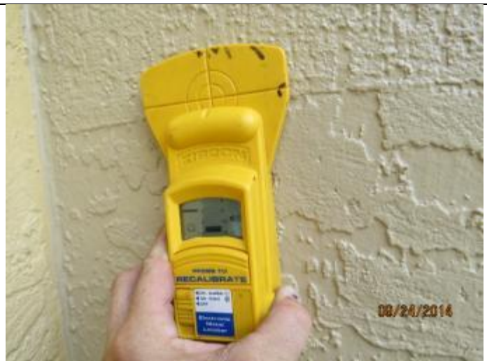
PHOTO 14 – Exterior Walls = Reinforced Masonry
