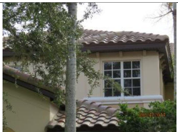
PHOTO 2 – Roof Overview, Covering = Tile
