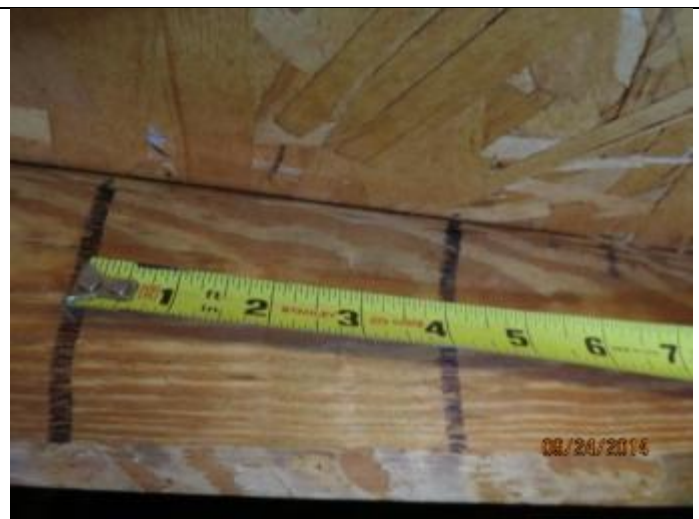
PHOTO 6 – Roof Deck Attachment Spacing
