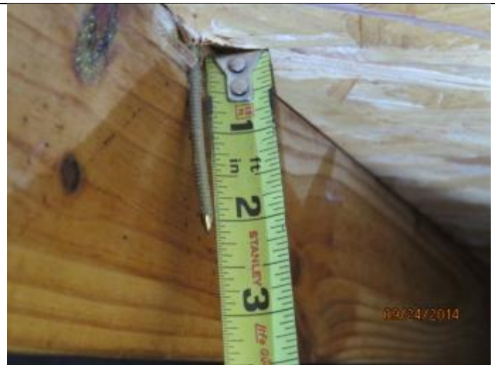
PHOTO 4 – Roof Deck Attachment = 8D Nails
