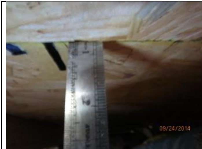
PHOTO 3 – Roof Deck = OSB
