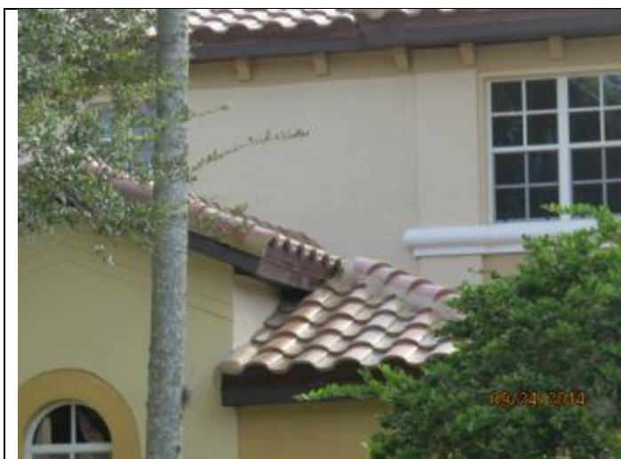
PHOTO 1 – Roof Overview, Covering = Tile
