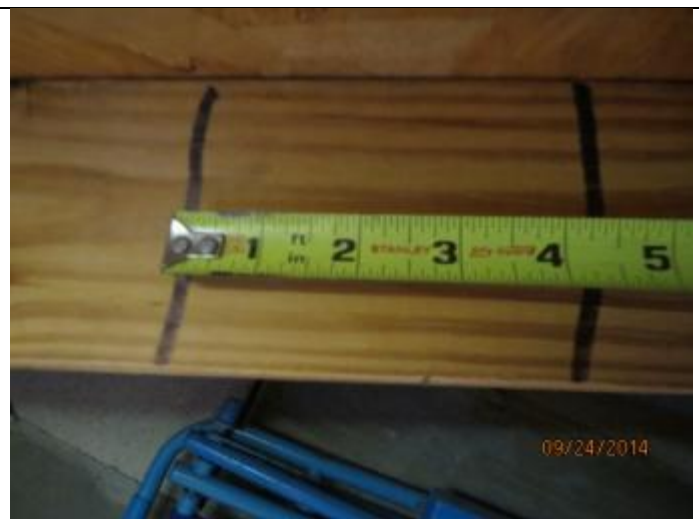
PHOTO 6 – Roof Deck Attachment Spacing
