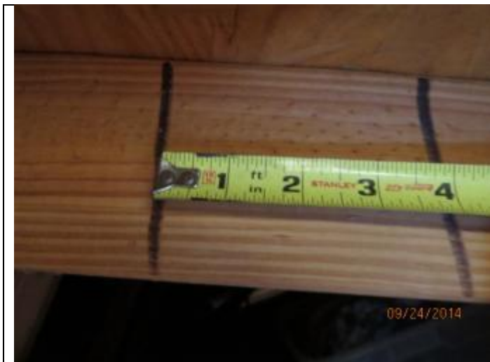
PHOTO 7 – Roof Deck Attachment Spacing
