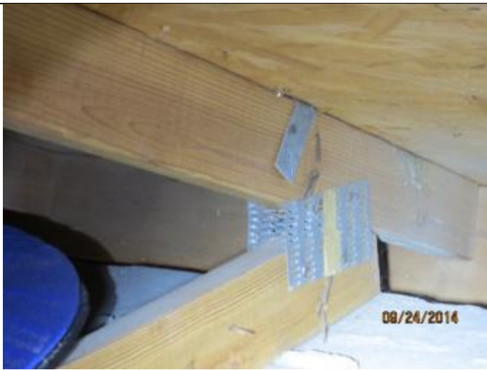
PHOTO 9 – Roof To Wall Attachment = Single Wrap Straps
