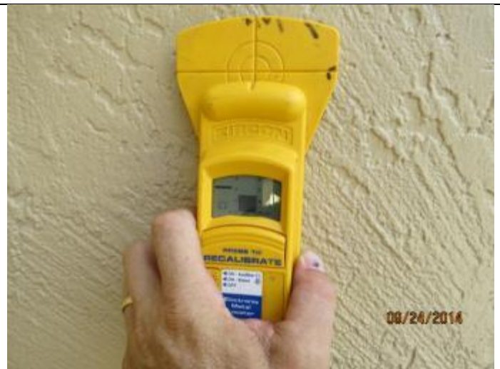
PHOTO 14 – Exterior Walls = Reinforced Masonry
