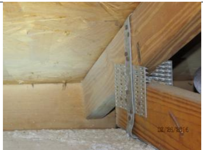
PHOTO 8 – Roof To Wall Attachment = Single Wrap Straps
