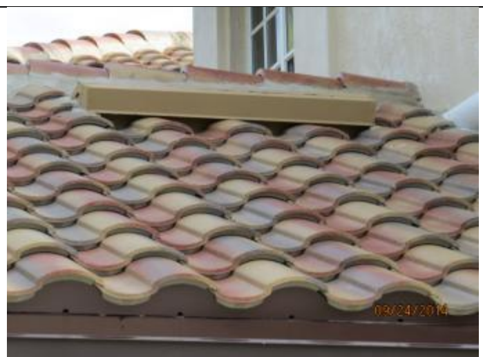
PHOTO 2 – Roof Overview, Covering = Tile
