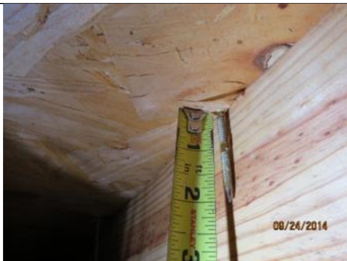
PHOTO 4 – Roof Deck Attachment = 8D Nails
