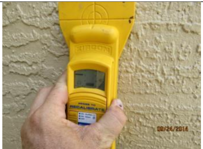
PHOTO 14 – Exterior Walls = Reinforced Masonry
