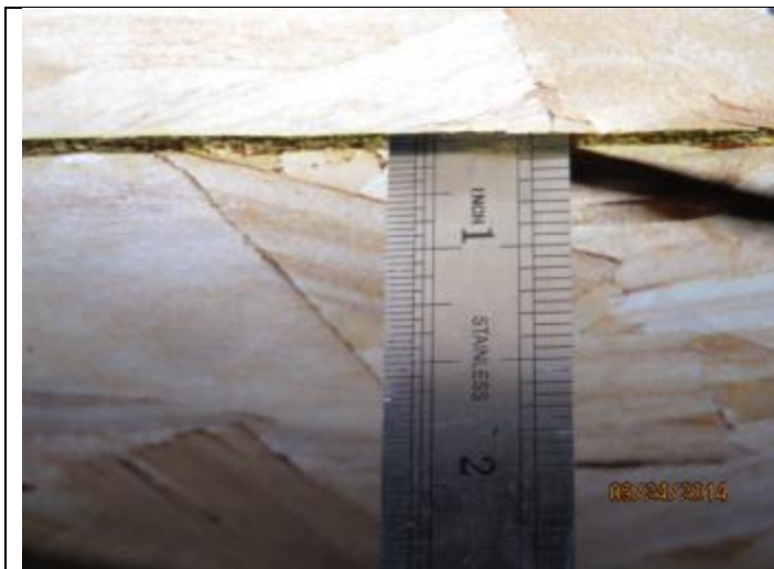
PHOTO 3 – Roof Deck = OSB
