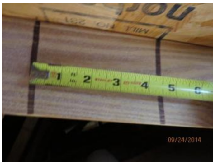
PHOTO 6 – Roof Deck Attachment Spacing
