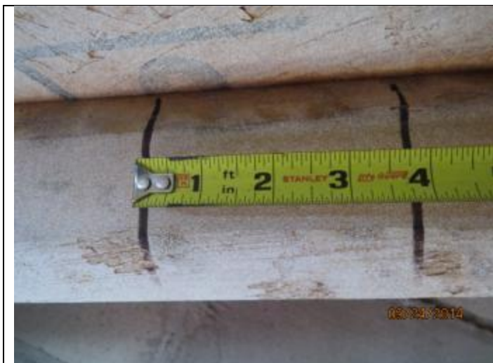
PHOTO 7 – Roof Deck Attachment Spacing
