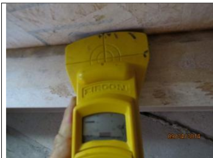
PHOTO 5 – Roof Deck Attachment Locations
