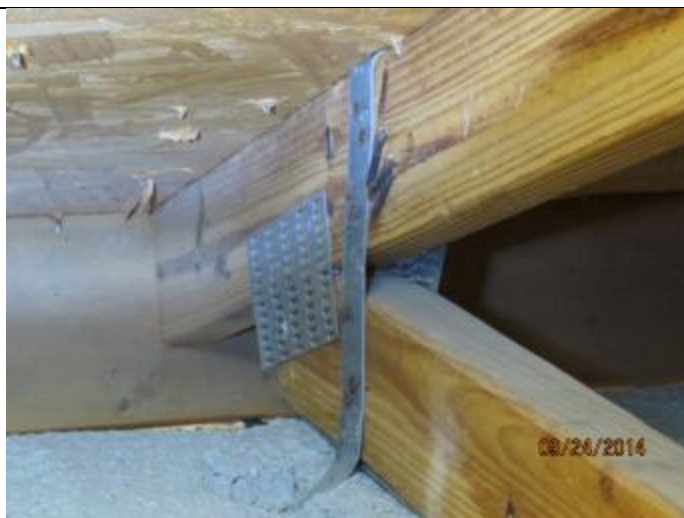
PHOTO 8 – Roof To Wall Attachment = Single Wrap Straps
