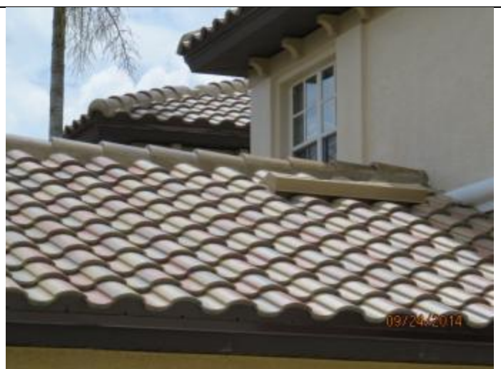
PHOTO 2 – Roof Overview, Covering = Tile
