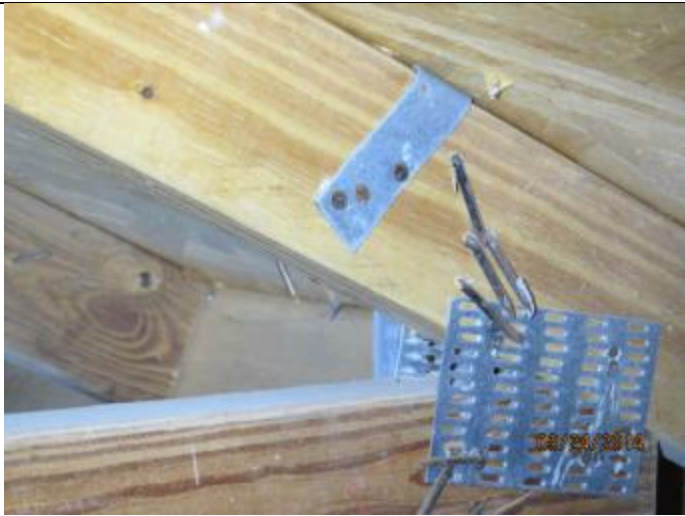
PHOTO 9 – Roof To Wall Attachment = Single Wrap Straps
