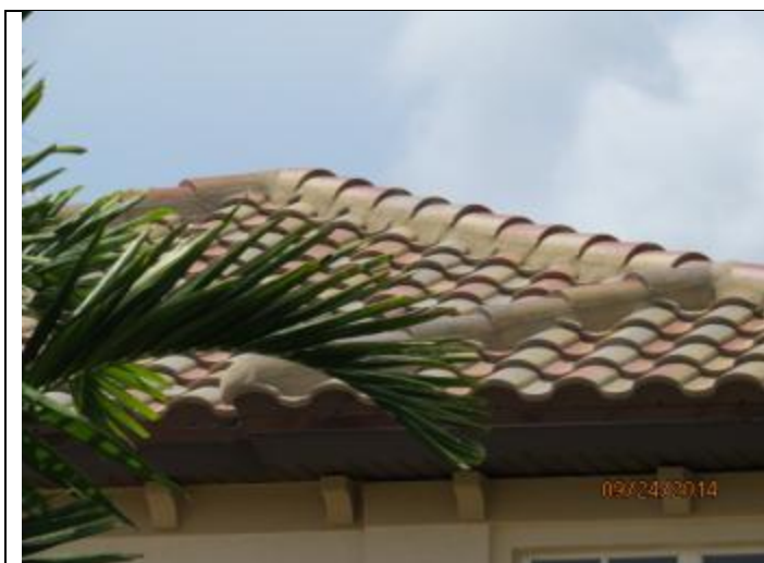
PHOTO 1 – Roof Overview, Covering = Tile
