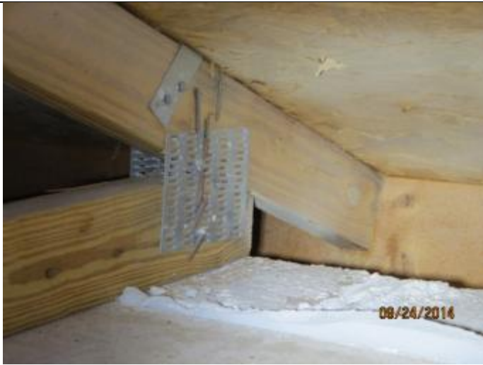
PHOTO 9 – Roof To Wall Attachment = Single Wrap Straps
