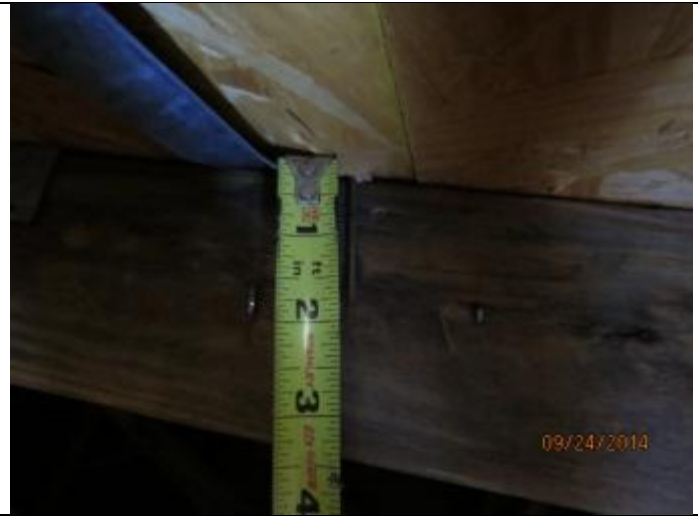
PHOTO 4 – Roof Deck Attachment = 8D Nails
