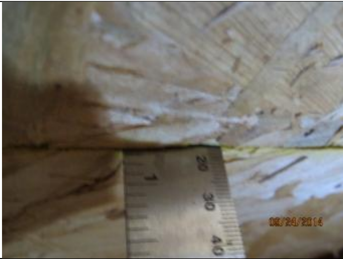
PHOTO 3 – Roof Deck = OSB
