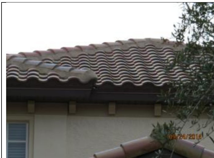
PHOTO 1 – Roof Overview, Covering = Tile
