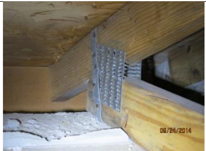
PHOTO 8 – Roof To Wall Attachment = Single Wrap Straps
