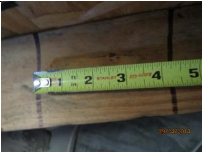
PHOTO 7 – Roof Deck Attachment Spacing
