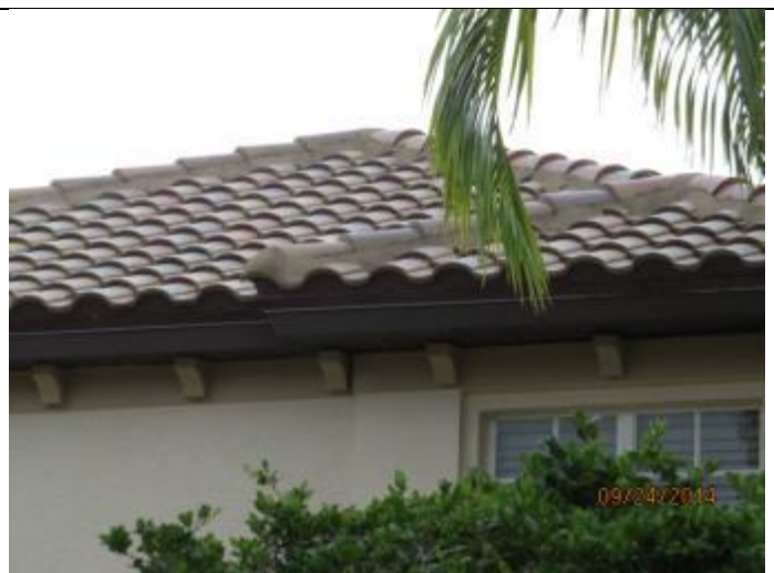
PHOTO 2 – Roof Overview, Covering = Tile
