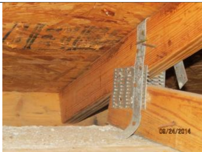
PHOTO 8 – Roof To Wall Attachment = Single Wrap Straps
