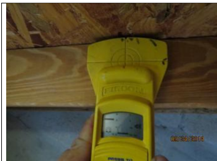
PHOTO 5 – Roof Deck Attachment Locations
