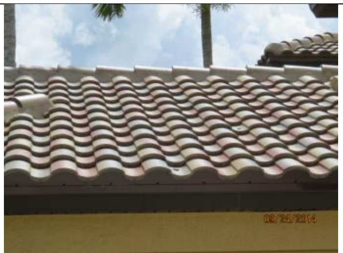
PHOTO 2 – Roof Overview, Covering = Tile
