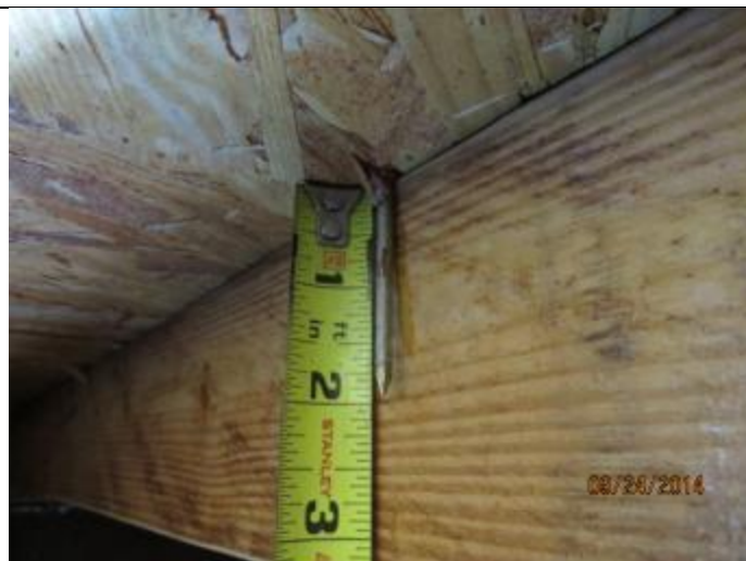
PHOTO 4 – Roof Deck Attachment = 8D Nails
