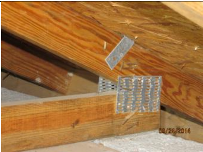
PHOTO 9 – Roof To Wall Attachment = Single Wrap Straps
