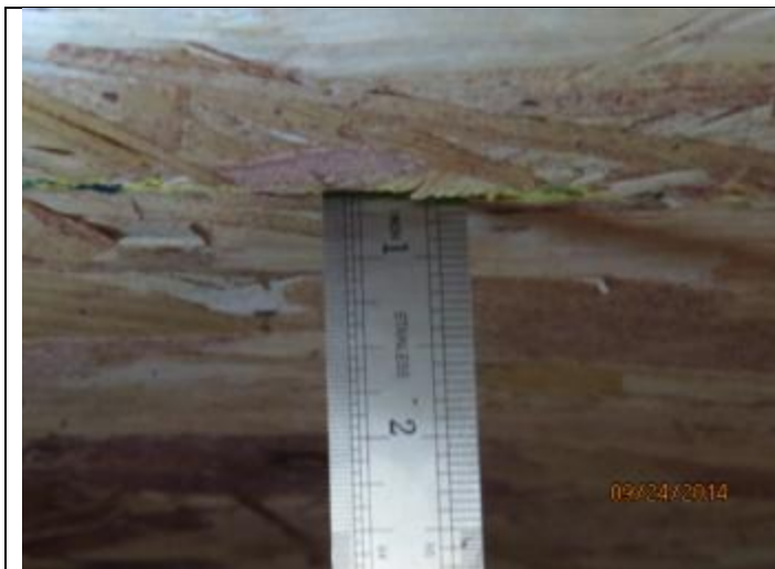
PHOTO 3 – Roof Deck = OSB
