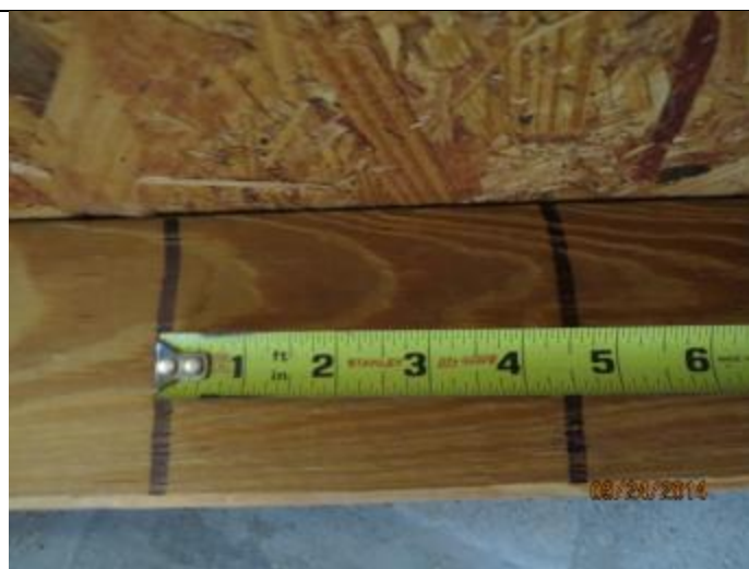
PHOTO 6 – Roof Deck Attachment Spacing
