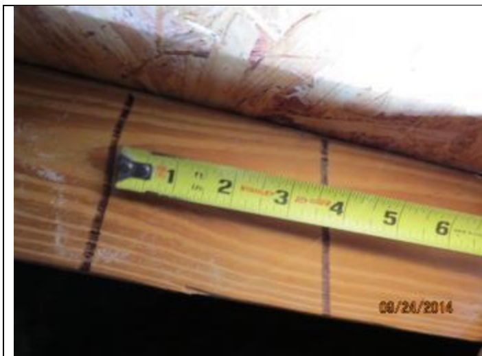
PHOTO 7 – Roof Deck Attachment Spacing
