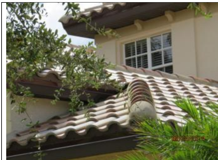
PHOTO 1 – Roof Overview, Covering = Tile
