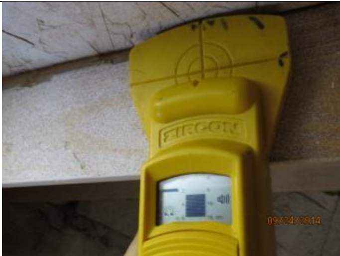
PHOTO 5 – Roof Deck Attachment Locations
