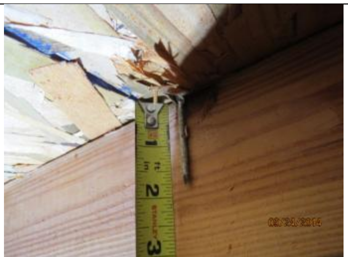
PHOTO 4 – Roof Deck Attachment = 8D Nails
