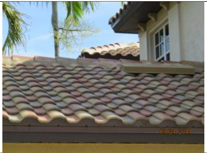
PHOTO 2 – Roof Overview, Covering = Tile
