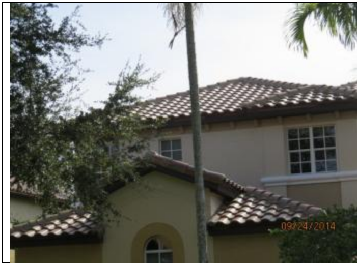
PHOTO 1 – Roof Overview, Covering = Tile
