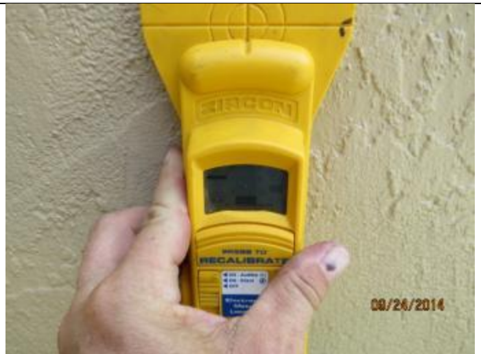
PHOTO 14 – Exterior Walls = Reinforced Masonry
