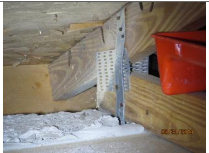
PHOTO 8 – Roof To Wall Attachment = Single Wrap Straps
