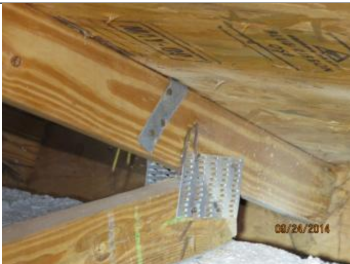
PHOTO 9 – Roof To Wall Attachment = Single Wrap Straps
