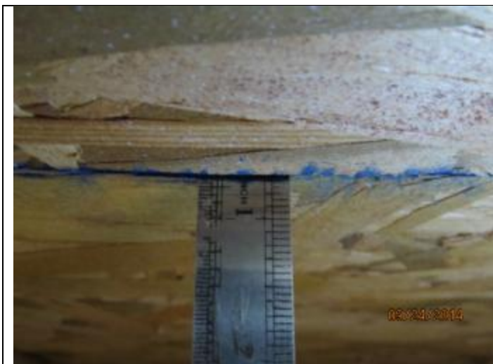
PHOTO 3 – Roof Deck = OSB
