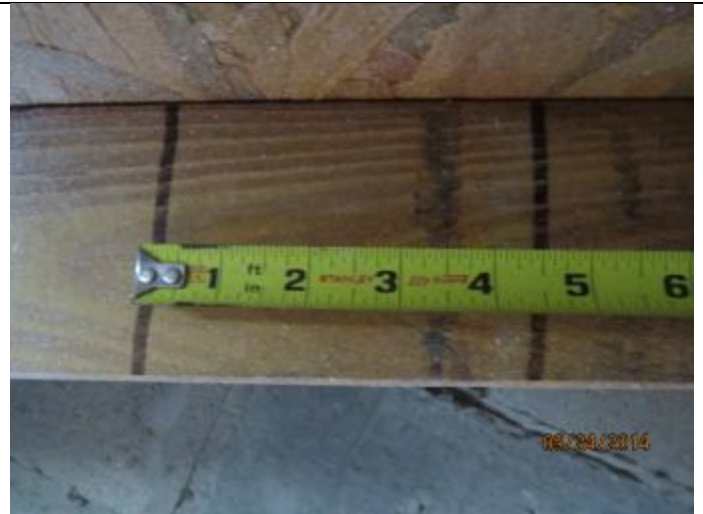
PHOTO 6 – Roof Deck Attachment Spacing
