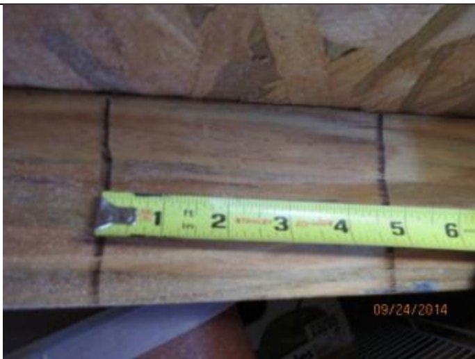
PHOTO 7 – Roof Deck Attachment Spacing
