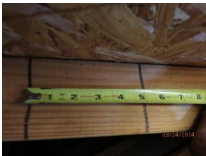
PHOTO 6 – Roof Deck Attachment Spacing
