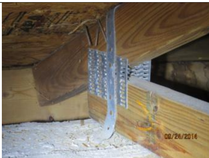
PHOTO 8 – Roof To Wall Attachment = Single Wrap Straps
