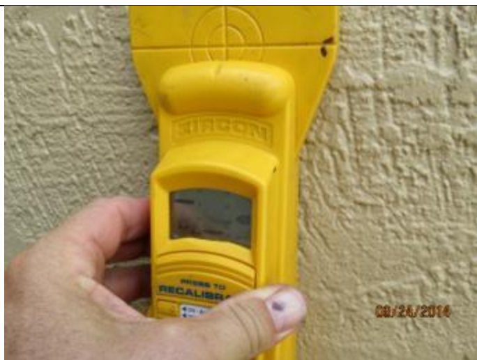
PHOTO 14 – Exterior Walls = Reinforced Masonry
