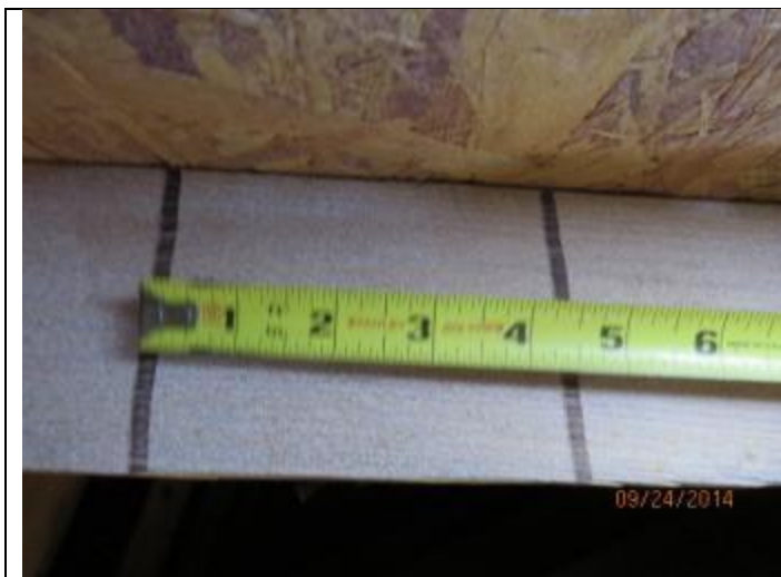
PHOTO 7 – Roof Deck Attachment Spacing
