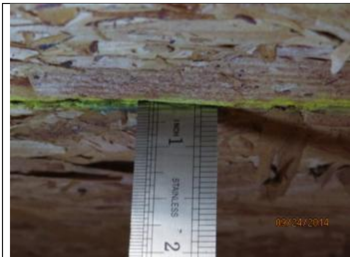
PHOTO 3 – Roof Deck = OSB
