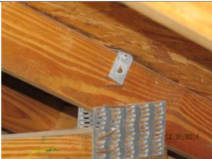
PHOTO 9 – Roof To Wall Attachment = Single Wrap Straps
