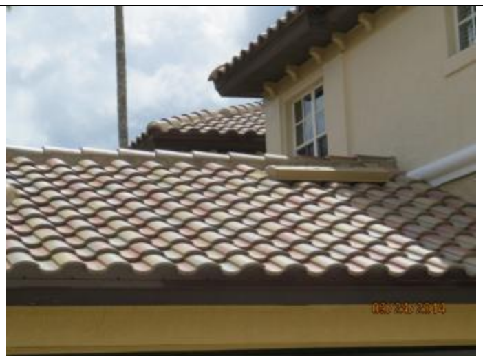
PHOTO 2 – Roof Overview, Covering = Tile
