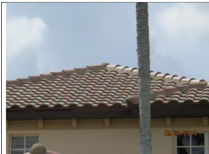
PHOTO 1 – Roof Overview, Covering = Tile
