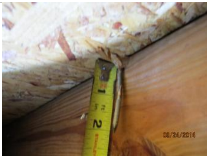
PHOTO 4 – Roof Deck Attachment = 8D Nails
