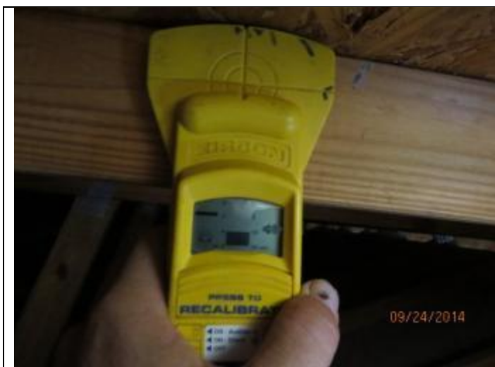
PHOTO 5 – Roof Deck Attachment Locations
