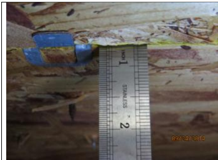
PHOTO 3 – Roof Deck = OSB
