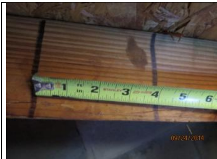
PHOTO 7 – Roof Deck Attachment Spacing
