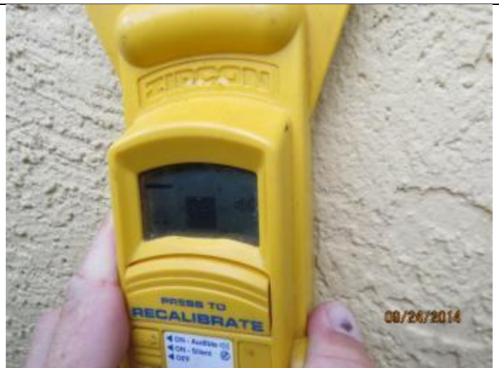
PHOTO 14 – Exterior Walls = Reinforced Masonry
