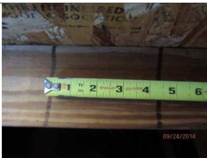
PHOTO 6 – Roof Deck Attachment Spacing
