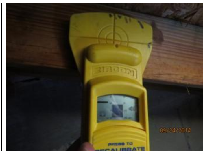
PHOTO 5 – Roof Deck Attachment Locations
