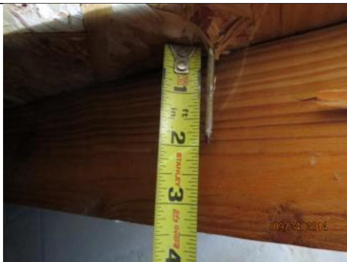
PHOTO 4 – Roof Deck Attachment = 8D Nails
