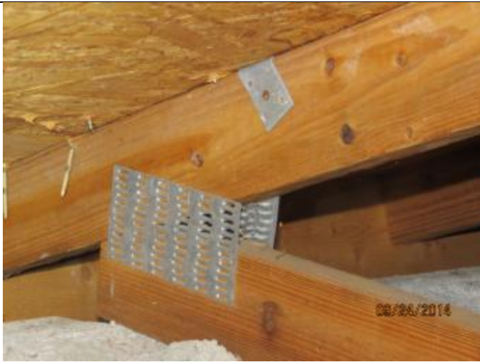
PHOTO 9 – Roof To Wall Attachment = Single Wrap Straps
