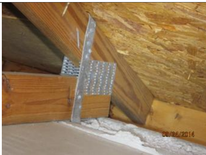
PHOTO 8 – Roof To Wall Attachment = Single Wrap Straps
