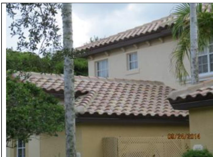
PHOTO 1 – Roof Overview, Covering = Tile
