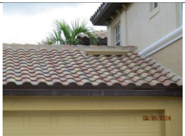
PHOTO 2 – Roof Overview, Covering = Tile
