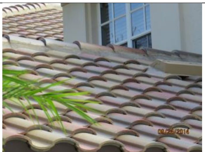
PHOTO 2 – Roof Overview, Covering = Tile
