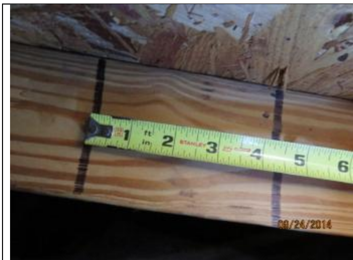
PHOTO 7 – Roof Deck Attachment Spacing
