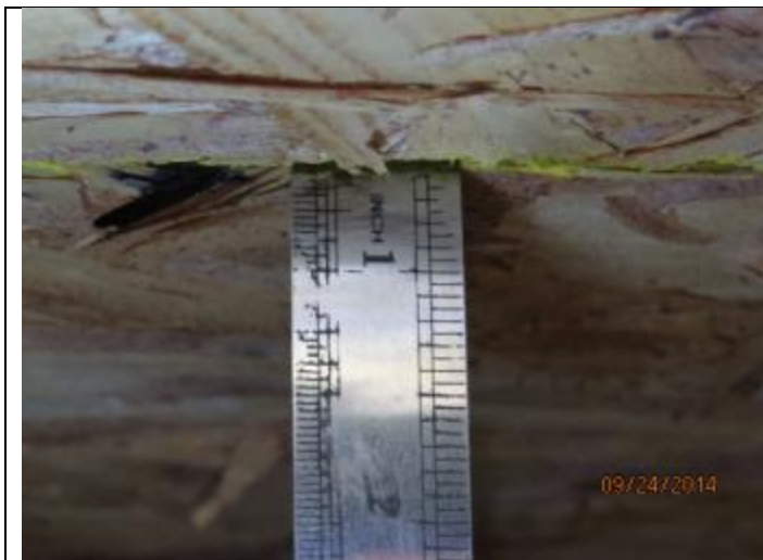
PHOTO 3 – Roof Deck = OSB
