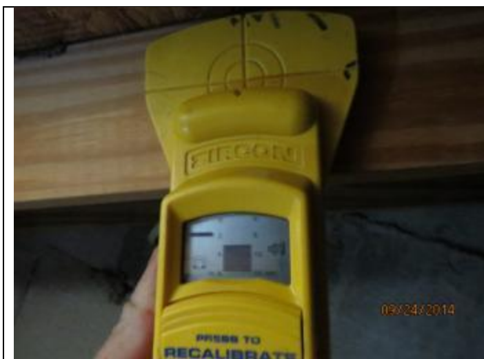
PHOTO 5 – Roof Deck Attachment Locations
