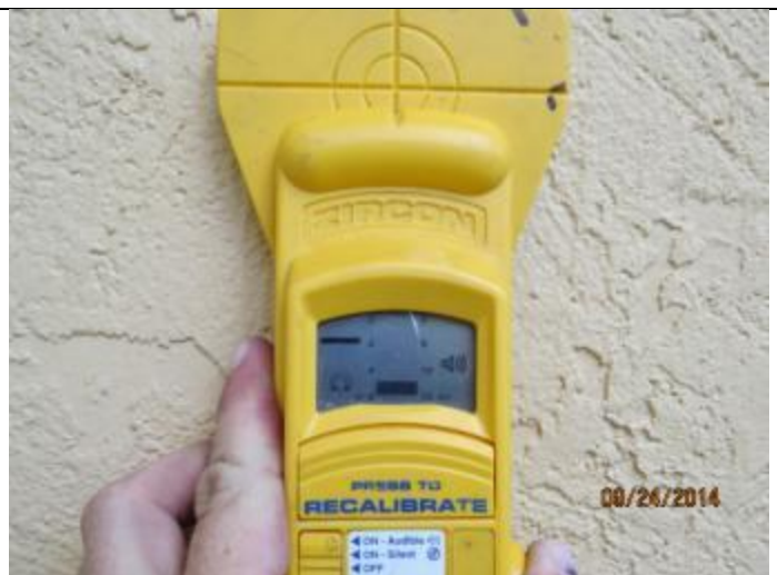
PHOTO 14 – Exterior Walls = Reinforced Masonry
