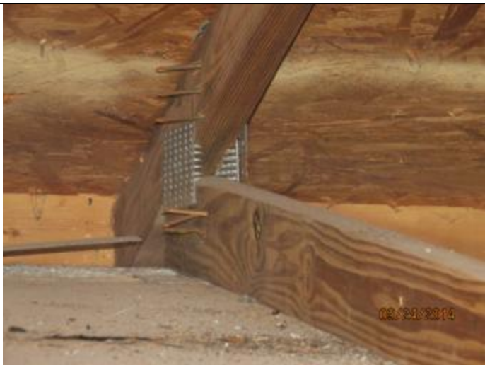
PHOTO 9 – Roof To Wall Attachment = Clips
