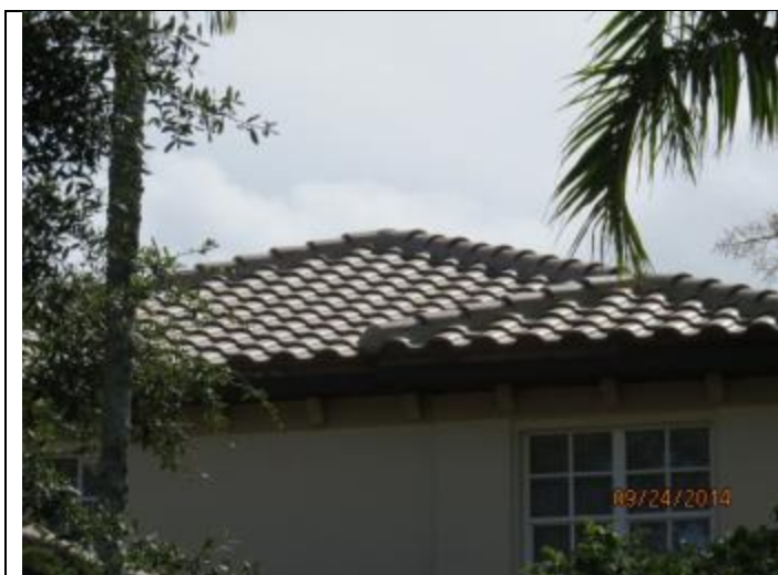
PHOTO 1 – Roof Overview, Covering = Tile
