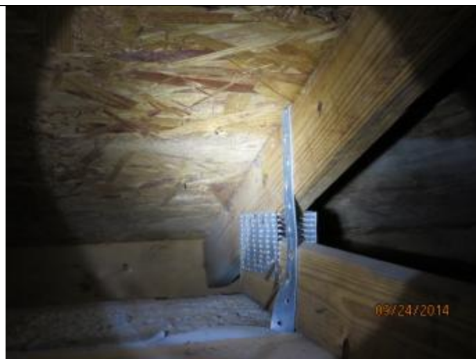
PHOTO 8 – Roof To Wall Attachment = Clips
