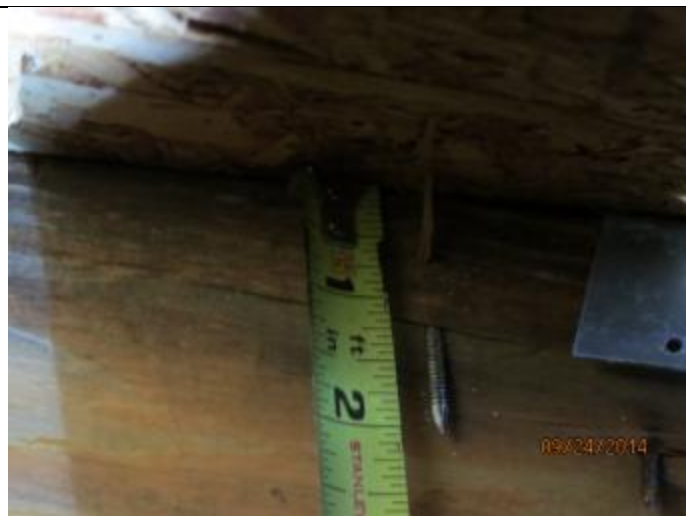
PHOTO 4 – Roof Deck Attachment = 8D Nails
