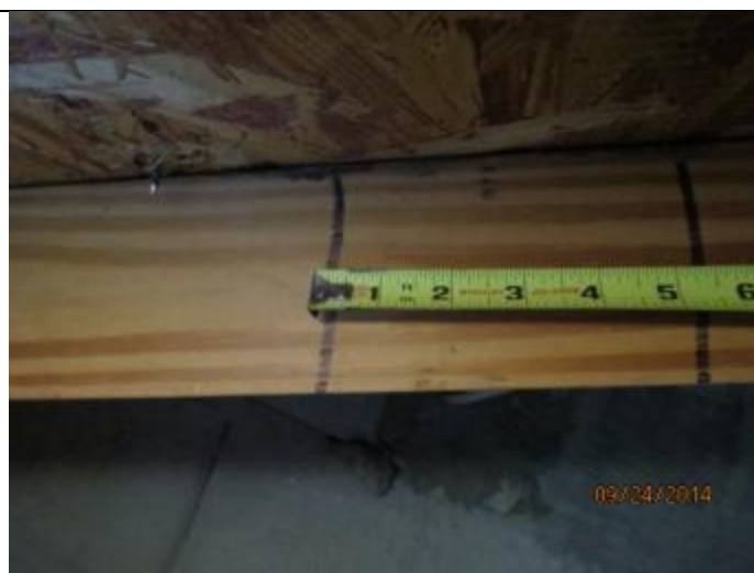
PHOTO 6 – Roof Deck Attachment Spacing
