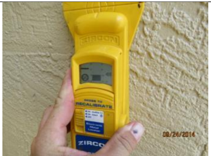
PHOTO 14 – Exterior Walls = Reinforced Masonry
