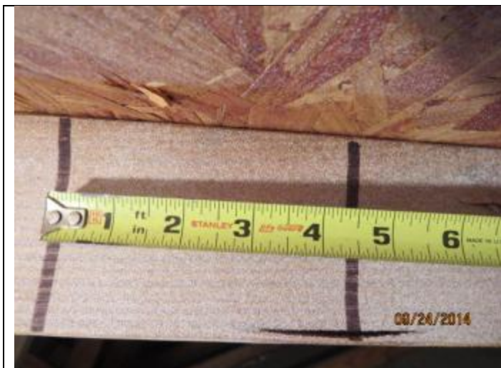
PHOTO 7 – Roof Deck Attachment Spacing
