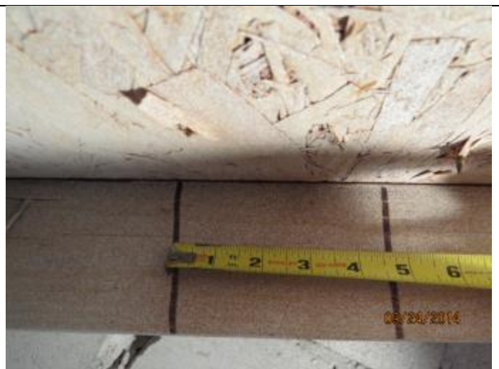
PHOTO 6 – Roof Deck Attachment Spacing
