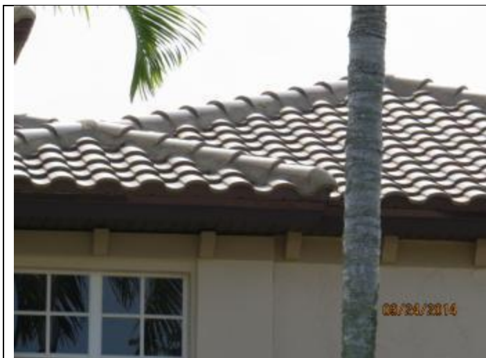
PHOTO 1 – Roof Overview, Covering = Tile
