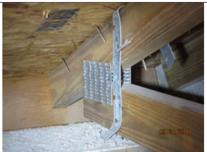
PHOTO 8 – Roof To Wall Attachment = Single Wrap Straps
