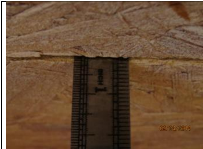
PHOTO 3 – Roof Deck = OSB
