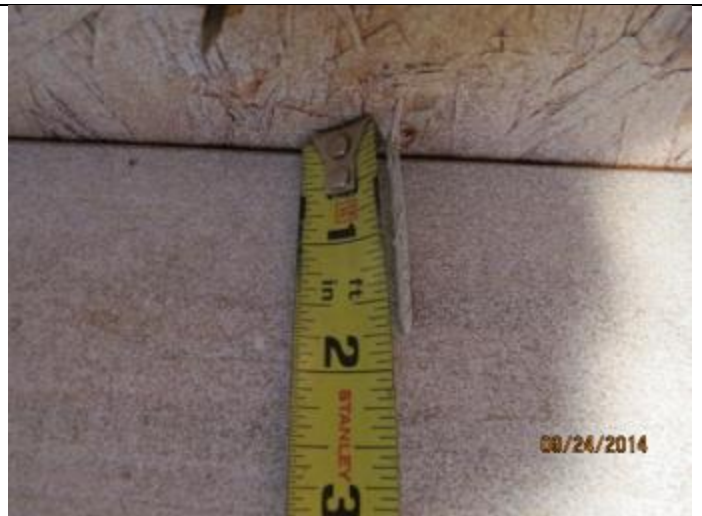
PHOTO 4 – Roof Deck Attachment = 8D Nails
