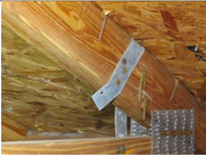
PHOTO 9 – Roof To Wall Attachment = Single Wrap Straps
