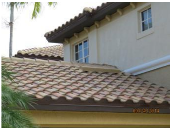
PHOTO 2 – Roof Overview, Covering = Tile
