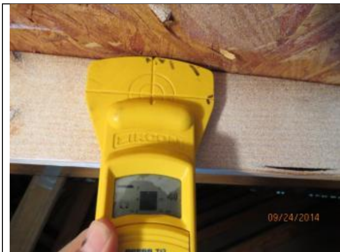
PHOTO 5 – Roof Deck Attachment Locations
