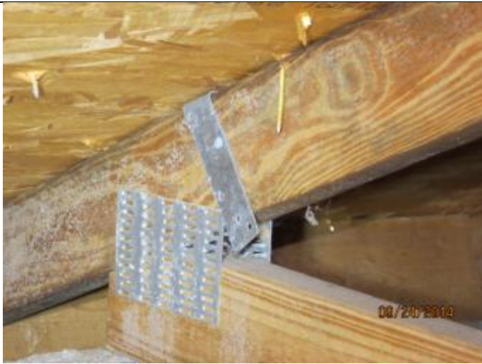
PHOTO 9 – Roof To Wall Attachment = Single Wrap Straps
