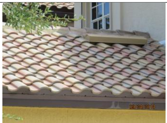
PHOTO 2 – Roof Overview, Covering = Tile
