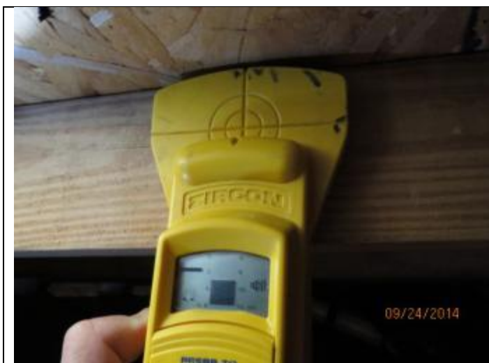
PHOTO 5 – Roof Deck Attachment Locations
