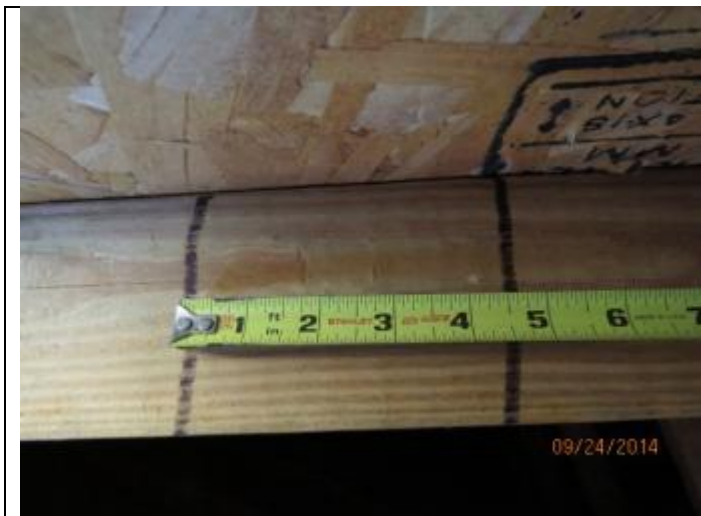
PHOTO 7 – Roof Deck Attachment Spacing
