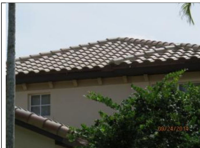
PHOTO 1 – Roof Overview, Covering = Tile
