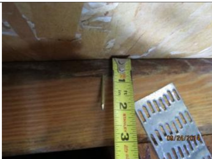
PHOTO 4 – Roof Deck Attachment = 8D Nails
