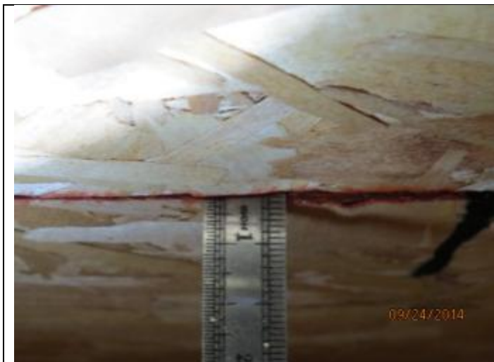
PHOTO 3 – Roof Deck = OSB
