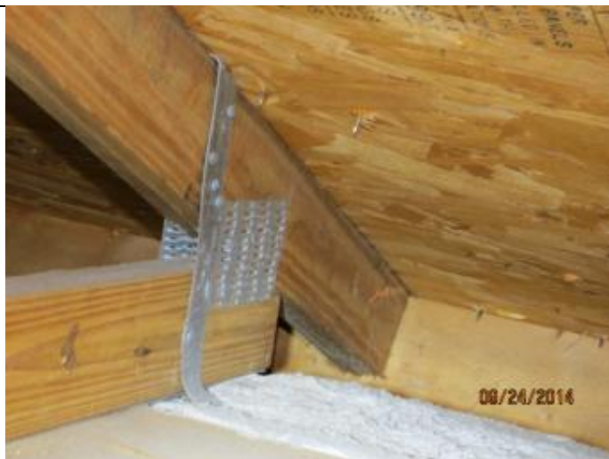
PHOTO 8 – Roof To Wall Attachment = Single Wrap Straps
