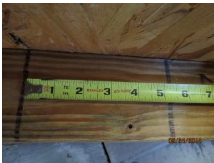
PHOTO 6 – Roof Deck Attachment Spacing
