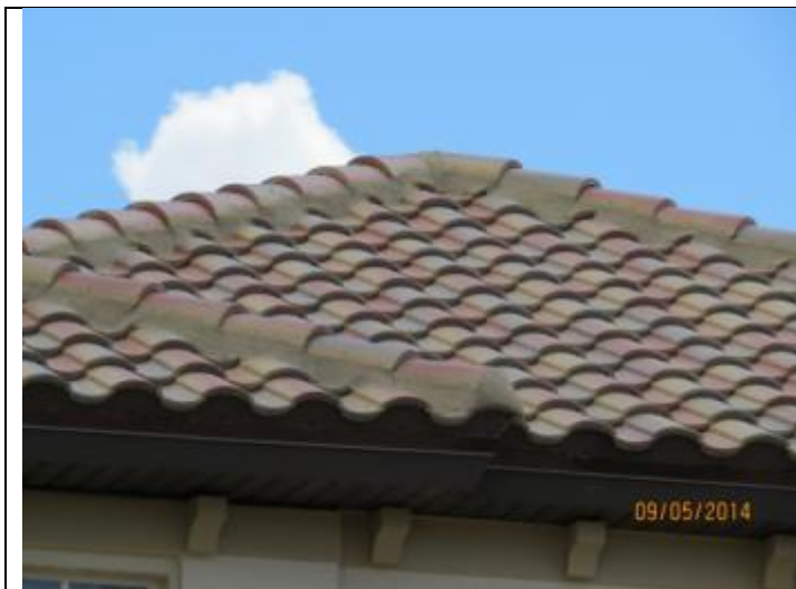
PHOTO 1 – Roof Overview, Covering = Tile
