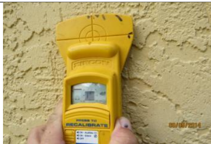
PHOTO 14 – Exterior Walls = Reinforced Masonry
