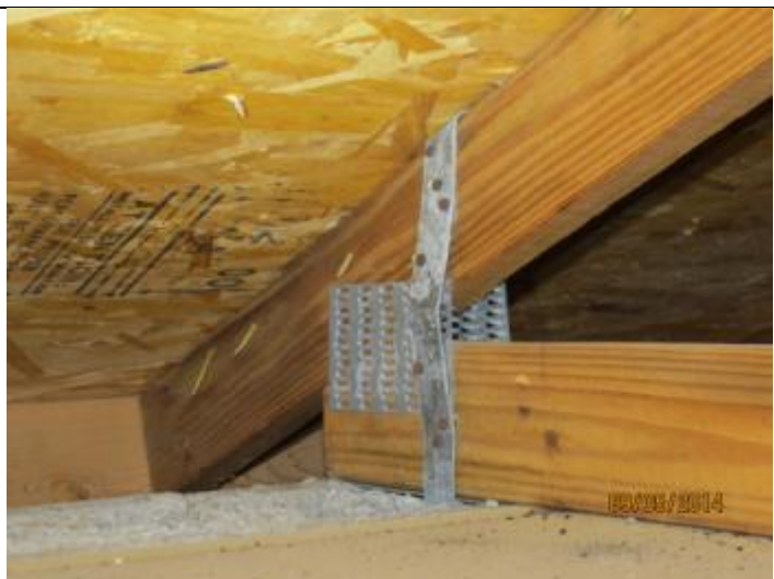
PHOTO 8 – Roof To Wall Attachment = Single Wrap Straps
