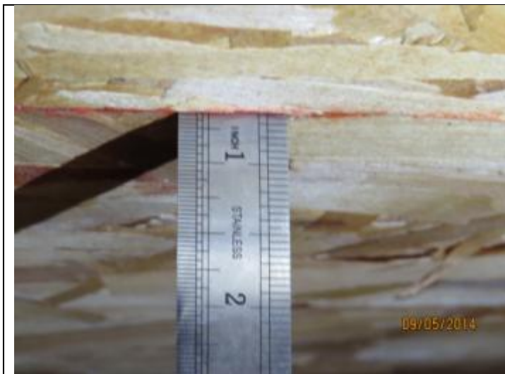
PHOTO 3 – Roof Deck = OSB
