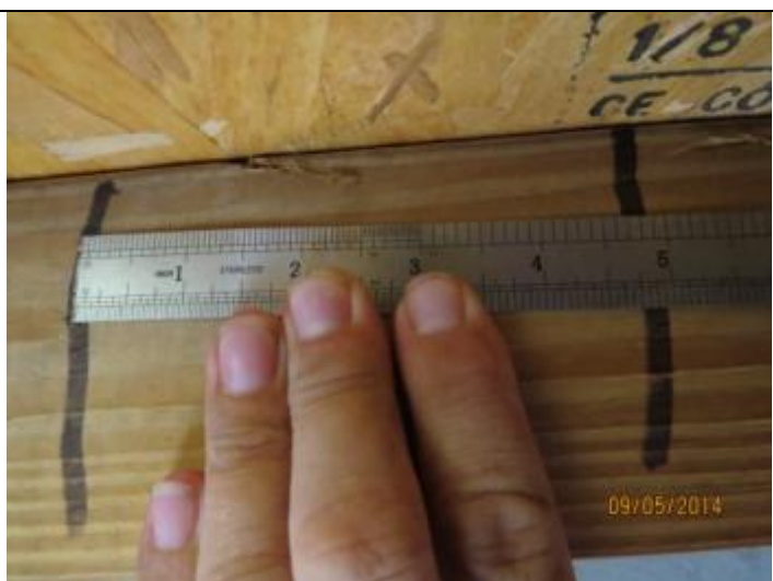
PHOTO 6 – Roof Deck Attachment Spacing
