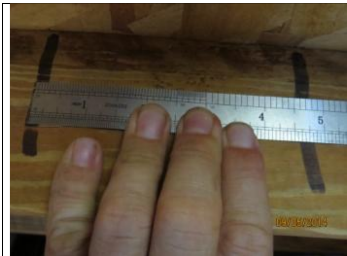
PHOTO 7 – Roof Deck Attachment Spacing
