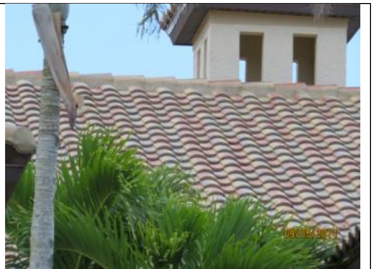
PHOTO 2 – Roof Overview, Covering = Tile
