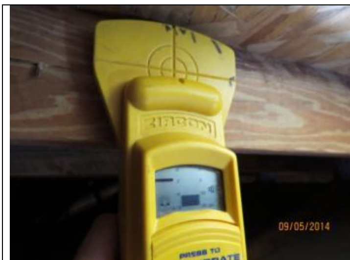
PHOTO 5 – Roof Deck Attachment Locations
