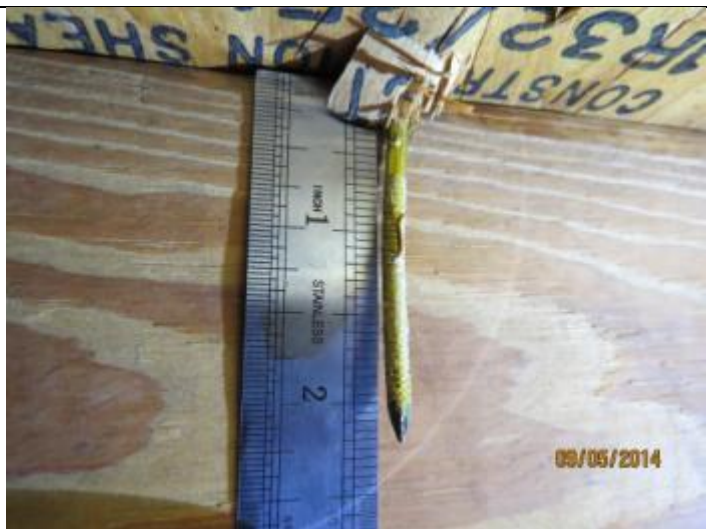
PHOTO 4 – Roof Deck Attachment = 8D Nails
