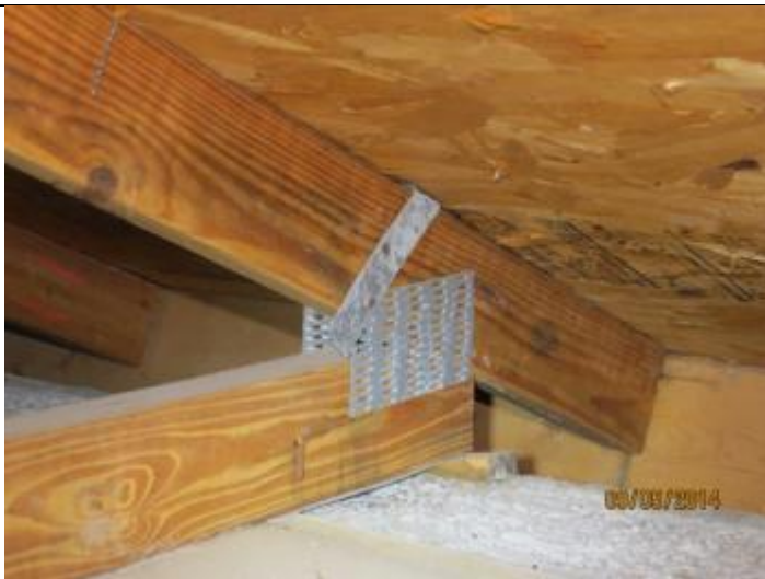
PHOTO 9 – Roof To Wall Attachment = Single Wrap Straps
