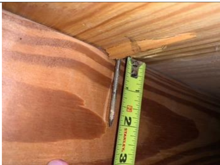
PHOTO 4 – Roof Deck Attachment = 8D Nails
