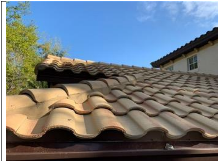
PHOTO 1 – Roof Overview, Covering = Tile
