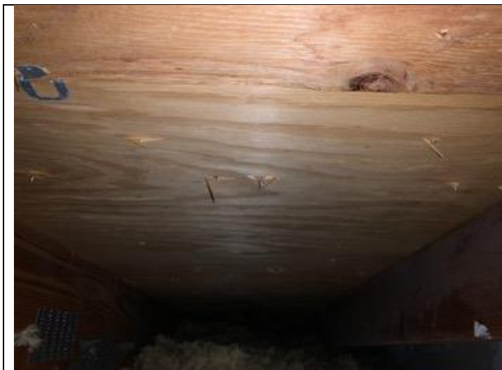
PHOTO 3 – Roof Deck = Plywood
