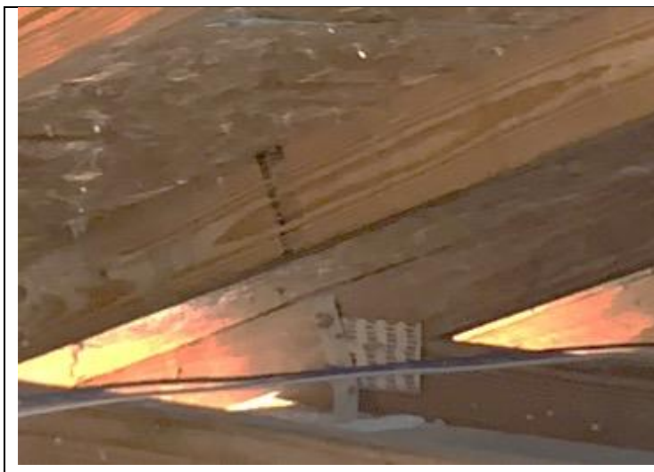
PHOTO 7 – Roof To Wall Attachment = Single Wrap Straps
