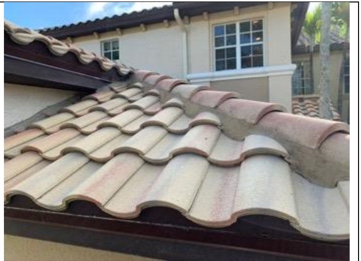
PHOTO 2 – Roof Overview, Covering = Tile
