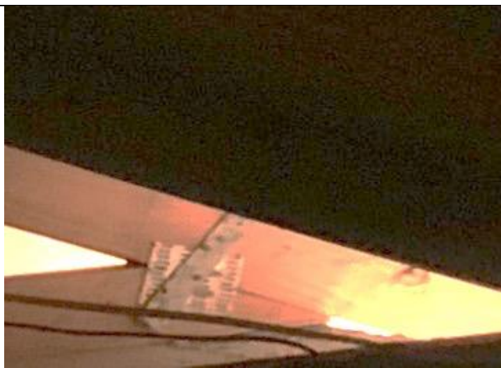
PHOTO 7 – Roof To Wall Attachment = Single Wrap Straps
