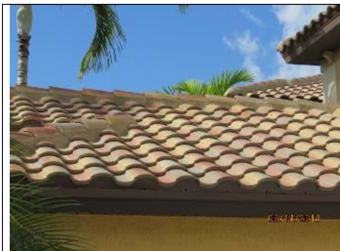
PHOTO 1 – Roof Overview, Covering = Tile
