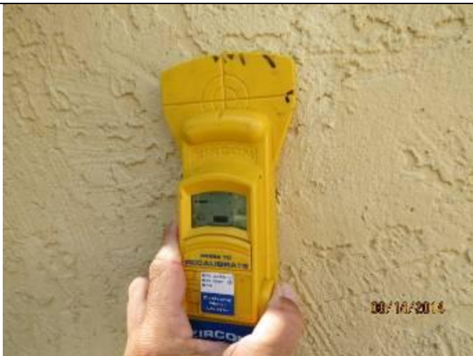
PHOTO 13 – Exterior Walls = Reinforced Masonry
