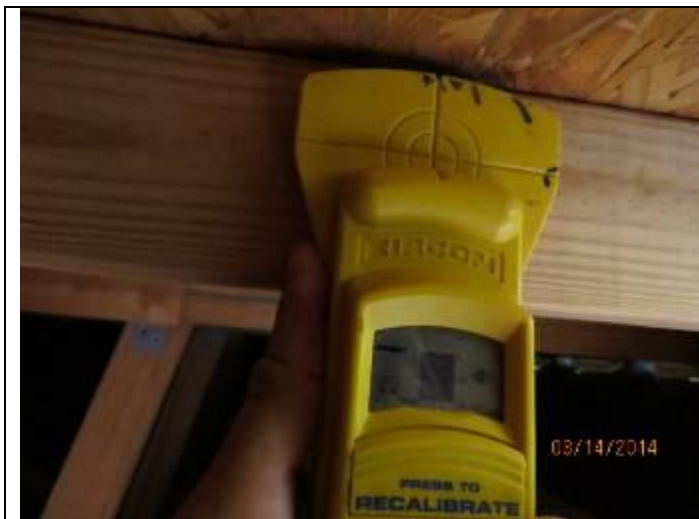
PHOTO 5 – Roof Deck Attachment Locations
