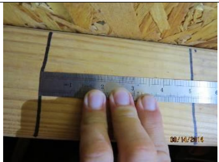
PHOTO 6 – Roof Deck Attachment Spacing
