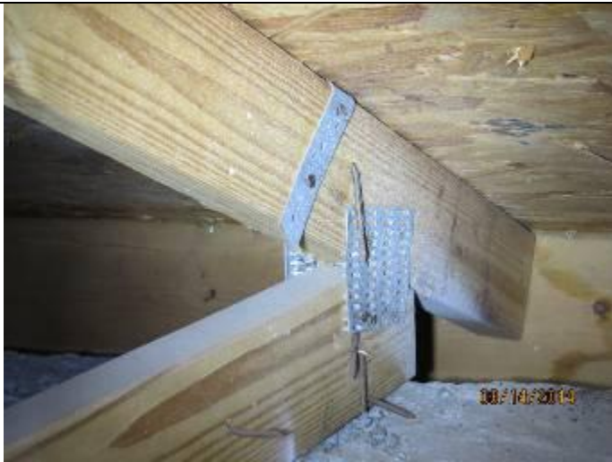
PHOTO 9 – Roof To Wall Attachment = Single Wrap Straps
