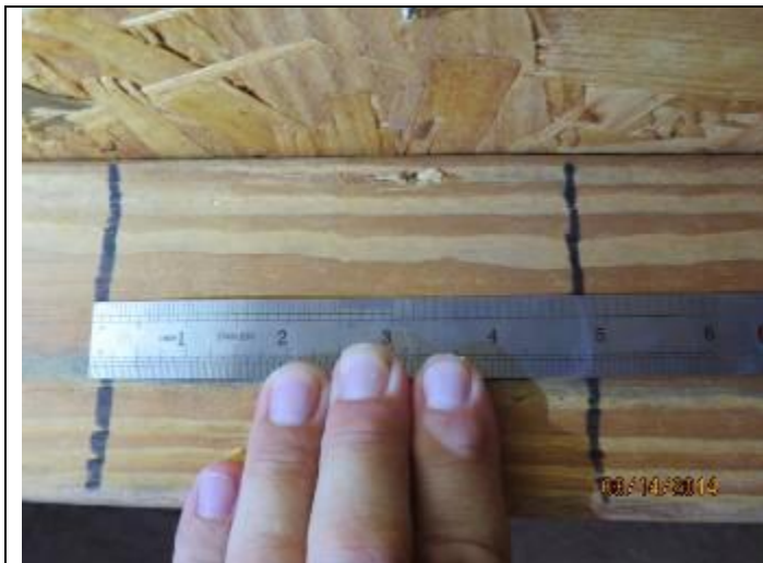
PHOTO 7 – Roof Deck Attachment Spacing
