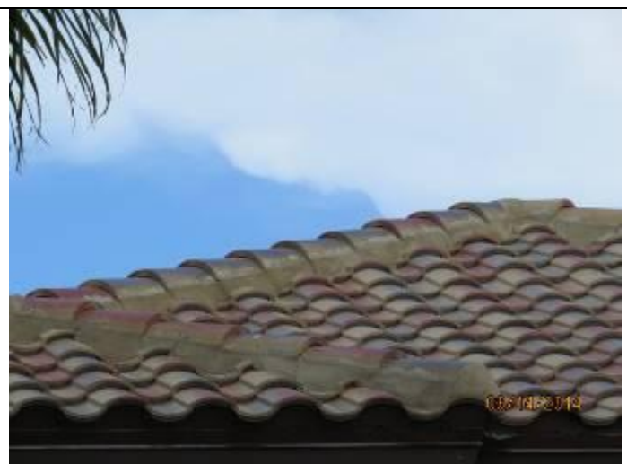
PHOTO 2 – Roof Overview, Covering = Tile
