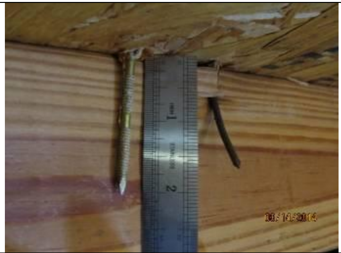
PHOTO 4 – Roof Deck Attachment = 8D Nails
