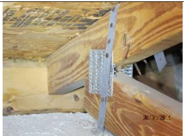
PHOTO 8 – Roof To Wall Attachment = Single Wrap Straps
